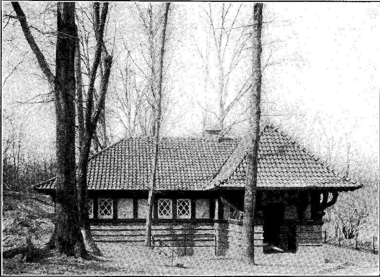
COMFORT STATION—NORTH MEADOW—CENTRAL PARK.
