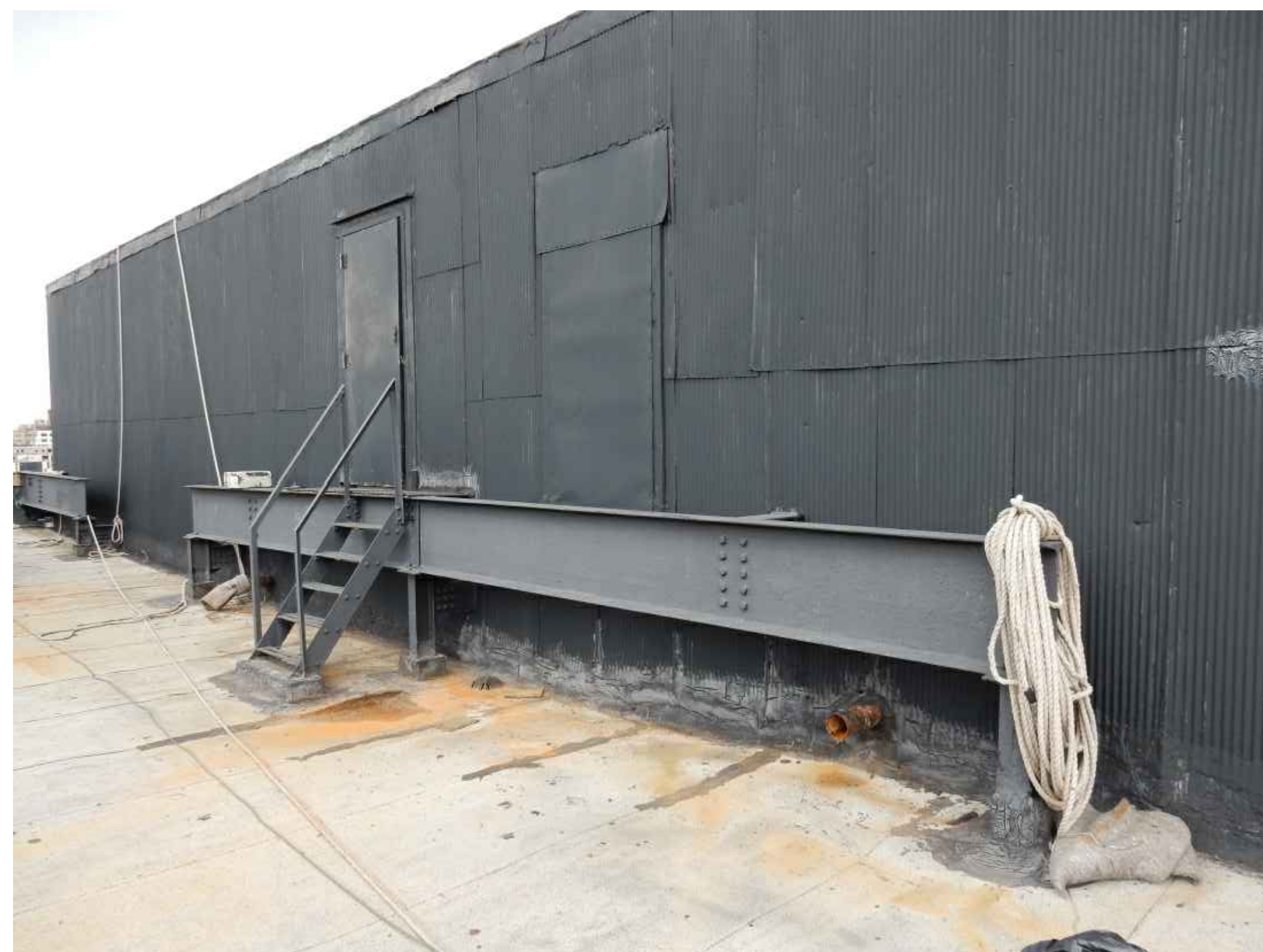
WATER TANK HOUSE LOOKING NORTHWEST
