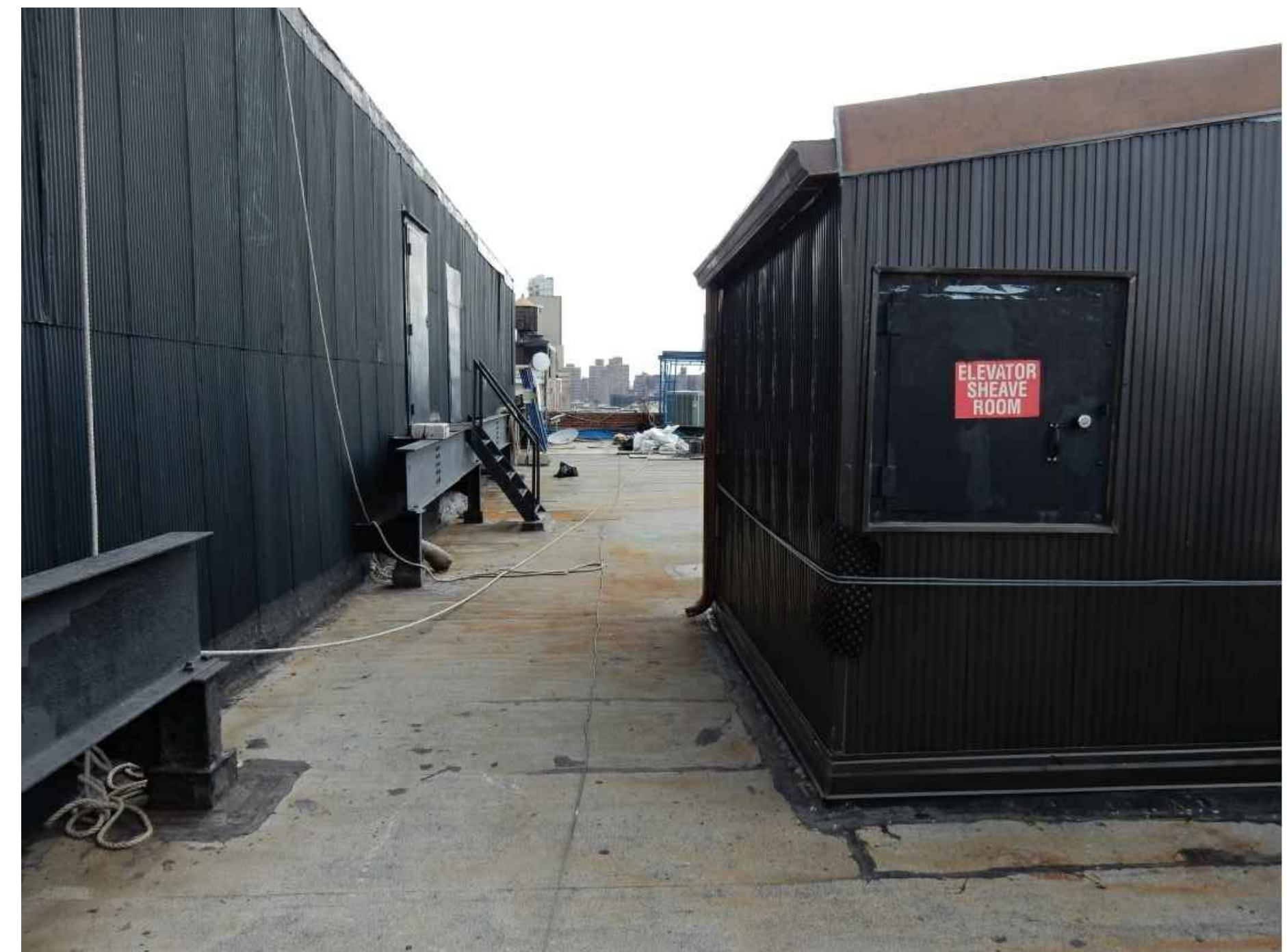
SOUTH ROOF LOOKING EAST
