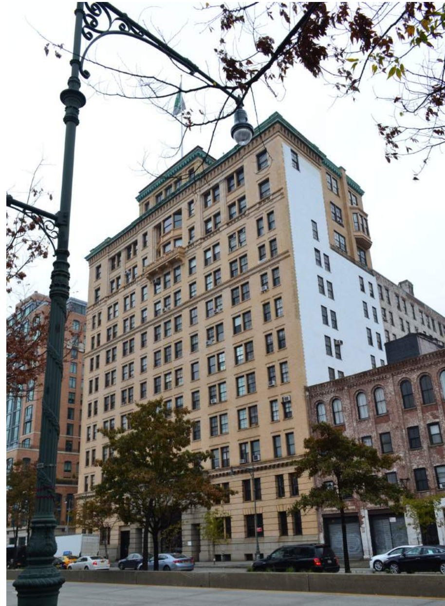
EXISTING FACADE FROM OF WEST STREET
