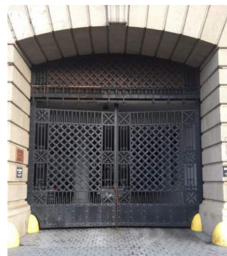
EXISTING DECORATIVE GATE - WEST STREET PASSAGEWAY
