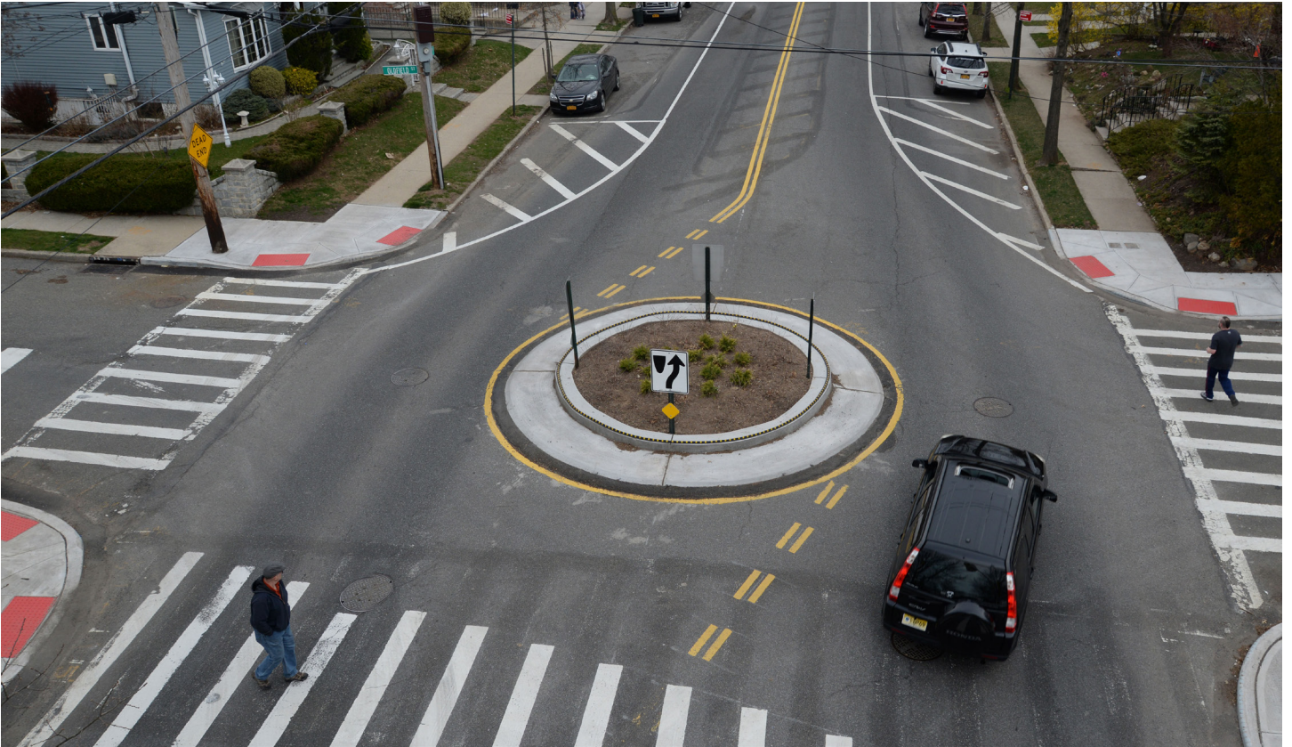
Neighborhood Traffic Circle: Greeley Avenue, Staten Island
