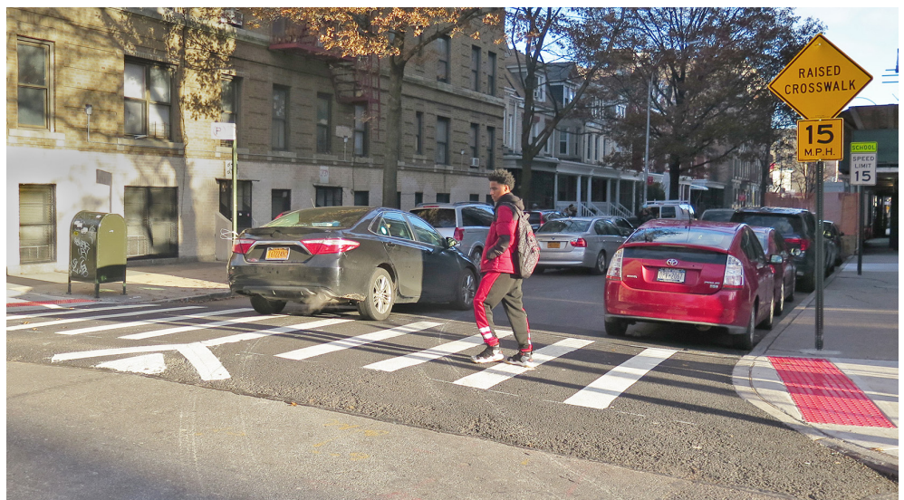
Raised Crosswalk: Briggs Avenue & East 196 Street, Bronx
