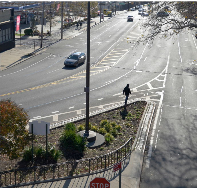
Street Improvement Project: Bay Street, Staten Island, Before
