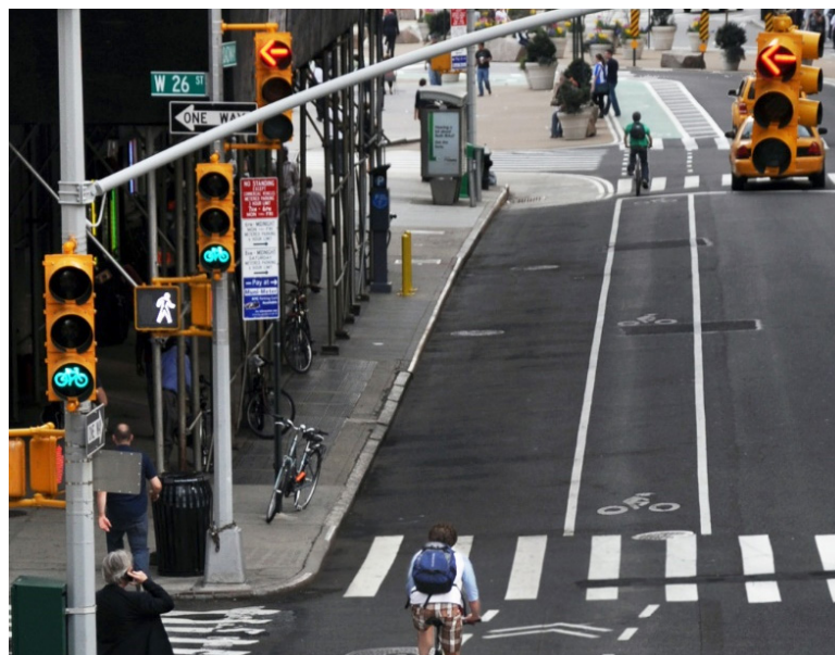
Turning Safety Signal Treatment: Broadway & 26 Street, Manhattan
