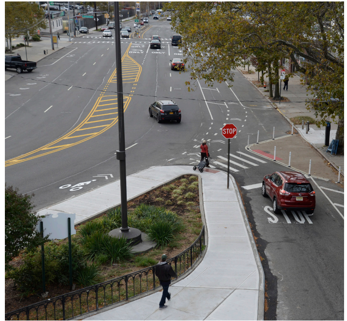
Street Improvement Project: Bay Street, Staten Island, After
