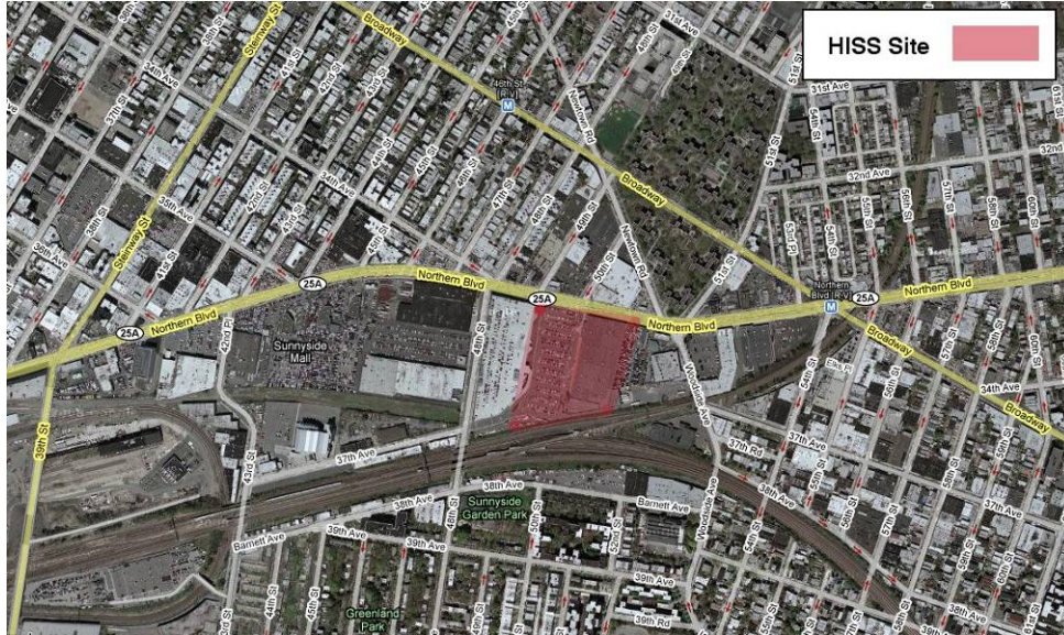
Figure 5: Aerial View of Northern Boulevard Facility
