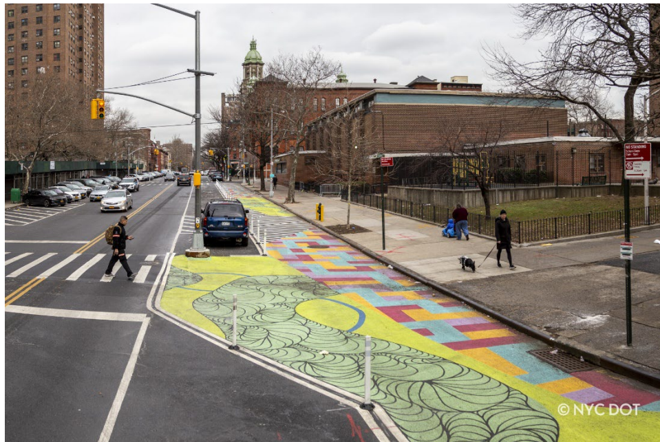
School Safety Project on Alexander Avenue in the Bronx
