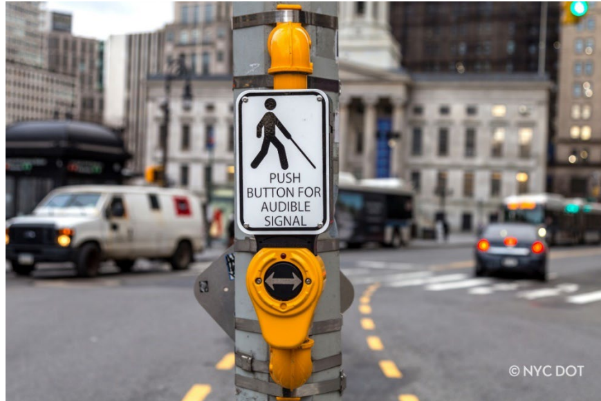
Accessible Pedestrian Signal at Court Street, Brooklyn
