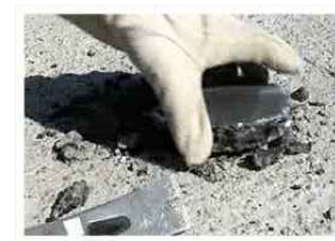
4. REMOVING SENSOR SHELL TOP
