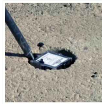
6. FILLING SENSOR HOLE WITH EPOXY
