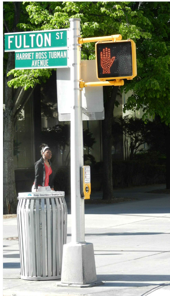
APS ON TYPICAL METAL POLE
