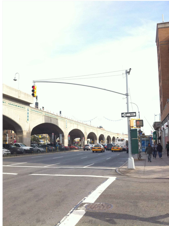
TRAFFIC SIGNAL ON "M-2A" POLE
