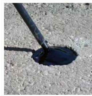
7. FILLING SENSOR HOLE WITH EPOXY UNTIL LEVELED WITH ROAD SURFACE
