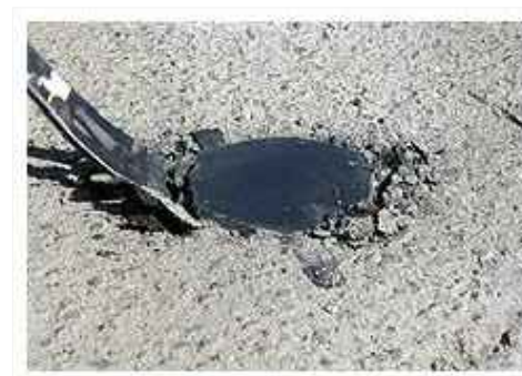
3. PRYING UPWARD TO LOOSEN SENSOR SHELL TOP
