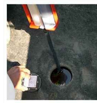
4. INITIAL EPOXY APPLICATION
