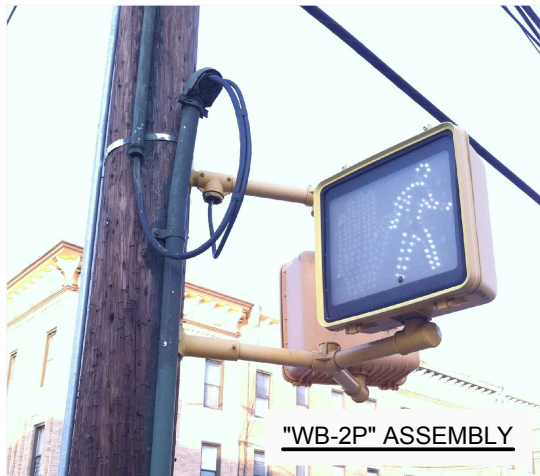
PEDESTRIAN SIGNALS ON WOOD POLE
