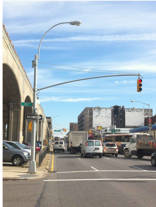
TRAFFIC SIGNAL ON "M-2A" COMBO POLE WITH 15-1/2" SHAFT EXTENSION
