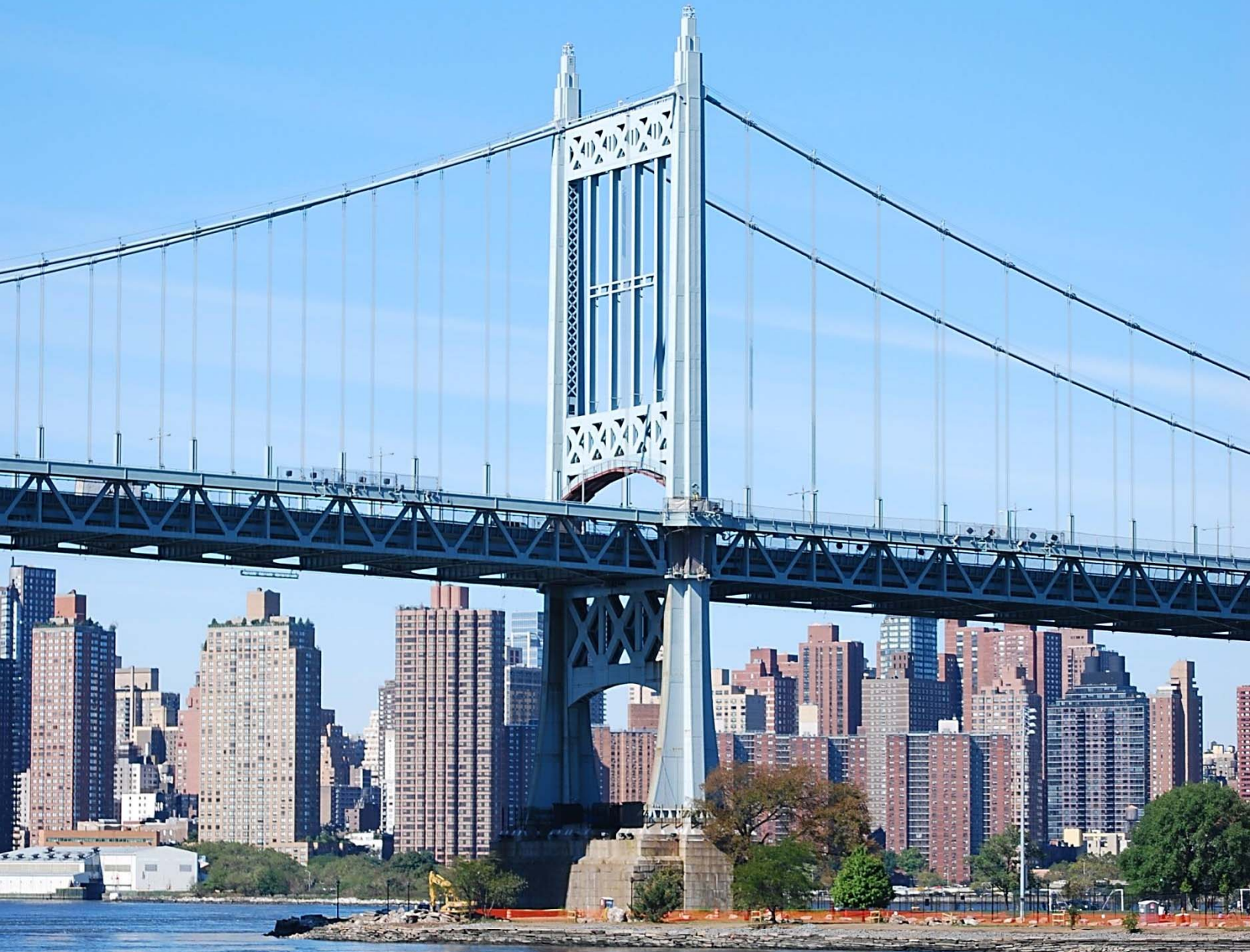
Robert F. Kennedy Memorial Bridge between Manhattan and Queens/Bronx
