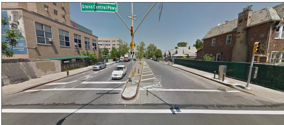
164th Street/Grand Central Pkwy SR N looking north
