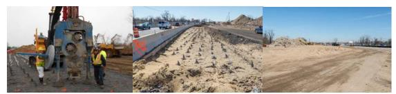
Northwest Quadrant Wick Drains for the New Mill Basin Bridge. Drains Backfilled.
