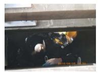
June 2018: Diver Installing a Splice Plate Underwater on the Belt Parkway over Gerritsen Inlet Bridge.
