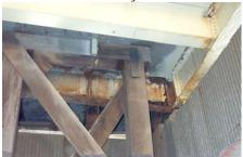
Timber Shoring Supporting a Failing Steel Beam - a Potential Winter Hazard. (Credit: Bojidar Yanev)
