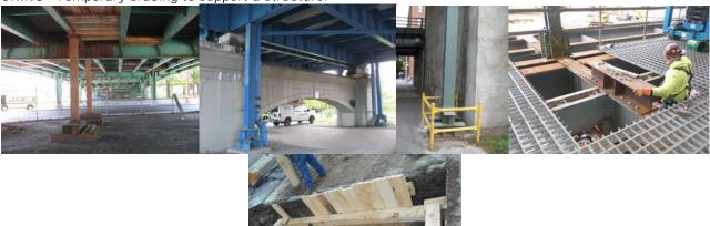
2014: Timber Shoring at Spans 7 and 8 of the Harlem River Drive over Ramp to and From Northbound Harlem River Drive. 2016: Steel Shoring at Span 5 of the East 174<sup>th</sup> Street Bridge over the Sheridan Expressway. Eastbound Brooklyn-Queens Expressway over Washington Street – Shoring on the Right Side of the End Abutment. 2018: Roosevelt Avenue West Viaduct Span 10 – Shoring for Steel Column Repairs, and Forest Avenue Culvert over Crystal Avenue - Installed Timber Shoring and Sheeting.
