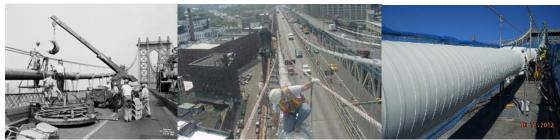
Replacing Cables on the Manhattan Bridge in 1955. (Credit: NYC Records) Inspector on Manhattan Bridge Cable.
