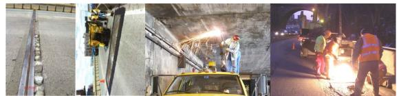
August 2014 PIA Safety Flag: Broken Joint Concrete Header and Steel Armor on the Long Island Expressway over Dutch Kills Creek. The Condition Was Made Safe By Installing Two Steel Plates. PIA Flag (Truck Wedged Under the FDR Drive at Span 41): Removing the Debris. (Credit: Victor Sandoval) PIA Flag Repair (Through Hole) on Harlem River Drive Ramp.
