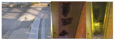
Example of PIA Safety Flag: Broken Grating. Chipping and Shielding at the Park Avenue Viaduct. Crew Removed Loose Concrete and Installed Expanded Sheet Metal Protective Shielding on the Underside of the Deck at Span #6.
