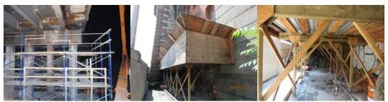
Old Mill Basin Bridge Scaffold Used During Pier Cap and Pier Column Repairs. 2019: Brooklyn Bridge Manhattan Approach, Arch Block A North Side - Overview of the Timber Scaffolding. View of the Underside of the Scaffolding.
