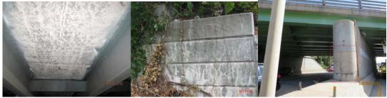
Union Street Bridge over Brooklyn-Queens Expressway in 2012 - Extensive Map Cracking With Efflorescence on the Underside of the Deck. (Credit: NYSDOT) Tompkins Avenue Bridge over B&O Railroad (Abandoned) in 2016 - Map Cracks With Efflorescence Near the End of the Wing Wall. Hamilton Place Bridge over Long Island Expressway in 2019 - Pier 1, Left Face of Stem.
