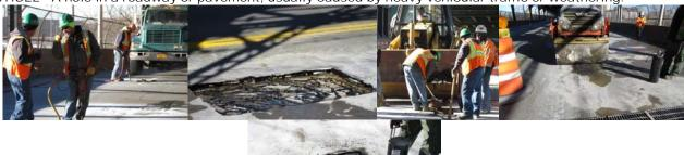
Repairing Potholes on the Roosevelt Avenue Bridge Deck Between Janet Place and 126th Street in January 2016. Each Perimeter is Sawcut. Filling in the Pothole With Asphalt. Paver Rolls Over the Pothole to Compact the Fill Material and Level the Surface. Finished Repair.
