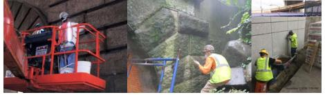
Pointing Joints on the East Face of the Brooklyn Anchorage of the Manhattan Bridge. Pointing the Masonry on the East Drive Bridge (East Wood Arch). 2018: Brooklyn Bridge Contract #6 - Ramp I - Pointing Joints.
