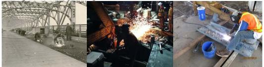
Welding I-Beam Locks on the Queensboro Bridge in 1938. (Credit: NYC Records) Welding Steel Packs for the Southbound Bruckner Expressway Bridge. June 2019: Roosevelt Avenue East Viaduct - Stage 2 – Welding Hex Nuts on the Back of Drain Boxes.
