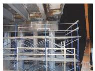
Mill Basin Bridge Scaffold Used During Pier Cap and Pier Column Repairs.
