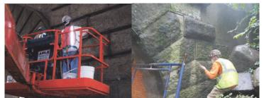
Pointing Joints on the East Face of the Brooklyn Anchorage of the Manhattan Bridge. Pointing the Masonry on the East Drive Bridge (East Wood Arch).
