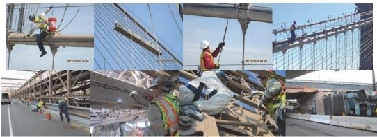
Brooklyn Bridge Contract #6 in 2014 - Painting Main Cables and Suspension Ropes. Painting at Main Bridge – Safety Barrier and Touchup. Containment at Ramp A, Span 4.
