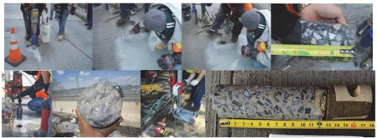
Removing a Core From 252<sup>nd</sup> Street Bridge over Henry Hudson Parkway in January 2009. (Credit: Masroor Mahmood) Core Sampling on the Bay Ridge Avenue Bridge in 2014. Utilizing a Coring Machine to Obtain a Concrete Core for Testing in June 2016 from the Westbound BQE over Adams Street.
