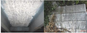
Union Street Bridge over Brooklyn-Queens Expressway in 2012 – Extensive Map Cracking With Efflorescence on the Underside of the Deck. (Credit: NYSDOT) Tompkins Avenue Bridge over B&O Railroad (Abandoned) in 2016 - Map Cracks With Efflorescence Near the End of the Wing Wall.
