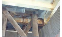
Timber Shoring Supporting a Failing Steel Beam - a Potential Winter Hazard. (Credit: Bojidar Yanev)
