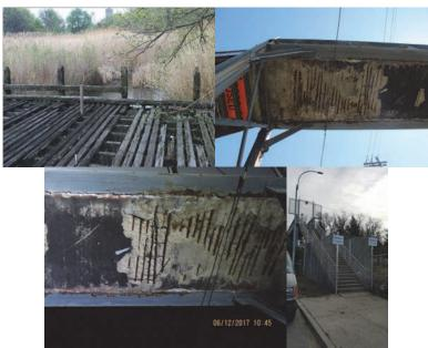
Flushing Meadow Park Pedestrian Bridge – (Date Unknown). 216<sup>th</sup> Street Pedestrian Bridge in April 2016: Delaminated Concrete and Detached Exposed Rebar at Span 4 – Deck Underside. June 2017 – Close-up of Span 4. Bridge Closed Sign.
