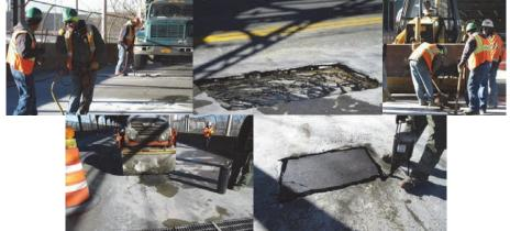
Repairing Potholes on the Roosevelt Avenue Bridge Deck Between Janet Place and 126th Street in January 2016. Each Perimeter is Sawcut. Filling in the Pothole With Asphalt. Paver Rolls Over the Pothole to Compact the Fill Material and Level the Surface. Finished Repair.
