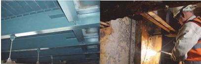
Stringers on the Manhattan Bridge. (Credit: NYSDOT) Bridge Repairer and Riveter Joseph Antony Repairing a Red-Flagged Stringer on the Bridge. (Credit: Hany Soliman)
