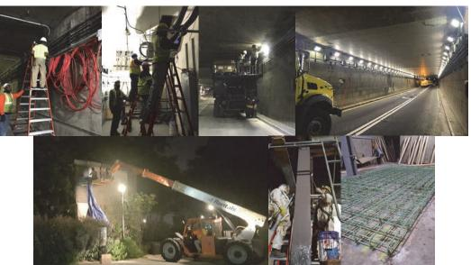
Battery Park Underpass – June and November 2017 – Installation of Cables and Conduits. January and July 2017: Lighting Fixture Repairs. August 2017: Surface Preparation for Turning Vane Painting. Intumescent Painting Application. October 2017 – Placement of Reinforcement for the New Fans' Bases. (Credit: Darlyn Alvarez)
