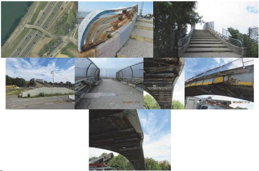
17<sup>th</sup> Avenue Bridge – October 2016: Beginning Approach, Left Side – Extensive Corrosion on the Guide Railing. 17<sup>th</sup> Avenue Bridge: September 2017 - End Approach Pavement has Cracks and Extensive Scaling. Corroded Guide Railing. Wearing Surface Exhibits Cracks and & Extensive Scaling With Exposed Aggregates. Spalled Area Under Deck With Timber Planks And Wire Mesh. Span 1 Left and Right Side -Damaged Girders, due to Previous Impacts.
