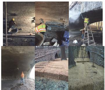
April 2017: Installing the New Underside Bricks - Matching Bricks in Color and Dimensions. Power Washing Under the Arch. Erosion Control Material Placed Over the Bridge Slope.
