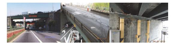
The joints at the multigirder bridges have deteriorated and the asphalt pavement exhibits alligator cracks and an uneven riding surface. Temporary supports have been placed at multiple locations to transfer the load from deteriorated bearings and/or bearing seats. The bridges have adequate load carrying capacity.
