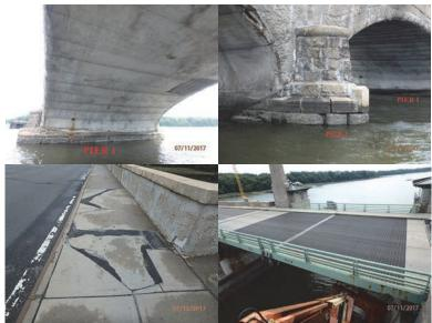
July 2017: Pier 1 Begin Face. Pier 2, Left End of Pier Nose - Typical Mortar Loss Between Stones. Span 6 Right Sidewalk Exhibits Full Width Shallow Spalls – Partially Patched by With Asphalt. Top of Span 4. (Credit: NYSDOT)
