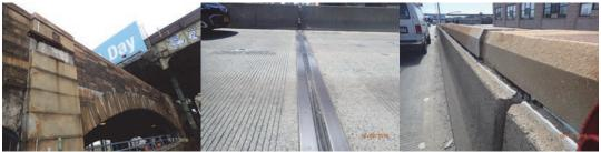
May 2016: Span 43, Right Side Fascia - the Stone Masonry Curtain Wall Exhibits Localized Moderate to Heavy Efflorescence Formation at Several Mortar Joints at the Outside Face and at the Underside of the Arch. Pier 19 Joint, Atlantic Avenue Westbound - Approximately 40% Length of Joint Compression Seal is Slightly Debonded. Spans 33 thru 35, Top of Deck, Right Fascia at Right Bridge Railing - Separation (up to 2") of the Fascia Stones From the Bridge Railing. (Credit: NYSDOT)
