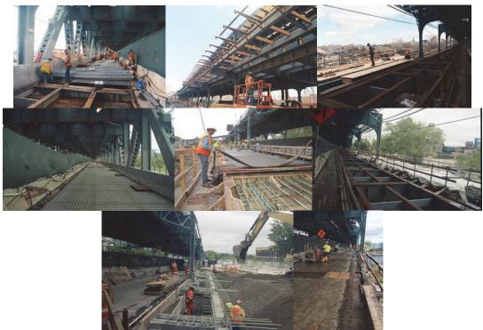
March 2017: Bascule Span - Installing Grid Deck for the Roadway. April 2017: West Viaduct – Formwork for the North Sidewalk. May 2017: Bascule Span Deck. West Viaduct – Stage 1 Sidewalk Test Panel Concrete Placement. West Approach – Stage 1 Sidewalk Preparation. East Viaduct – Stage 1 – Removing the Original Roadway Deck.
