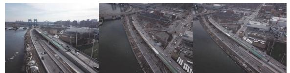
Drone Views: View South - Maintaining all Travel Lanes During Construction. View South From Above Bridge – Willis Avenue Bridge at Upper Left. View of Temporary Roadway for Northbound Traffic.
