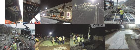
March 2017. Installing Stringers at Location #12. Through-Hole Repair.
