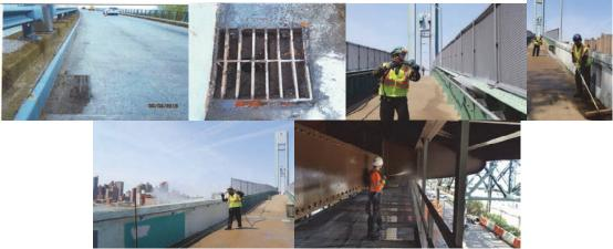
Debris and Sediment Fully Clogging a Scupper on the Northbound Roadway of the Boston Road Bridge over the Hutchinson River. Scupper After Cleaning. April 2016: Cleaning and Washing the Ward's Island Pedestrian Bridge. (Credit: Alaina Yuresko) May 2016: Washing the Underdeck of the Ed Koch – Queensboro Bridge. (Credit: Bojidar Yanev)
