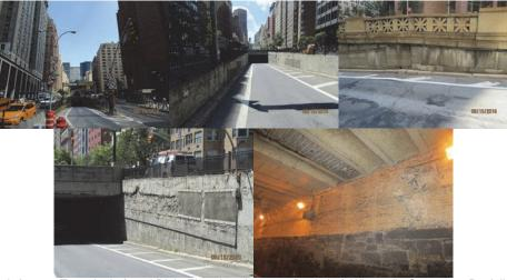
Park Avenue Tunnel – Left and Right Elevations in 2016. Begin Left Wingwall - Stones are Partially Dislodged, Cracked and With Missing Mortar. End Right Wingwall - Wall is Spalled and Exhibits Hollow Concrete Areas That are Shielded With Wire Mesh. End Abutment (Near South Portal) – Bricks Exhibit Deteriorated Mortar. (Credit: NYSDOT)
