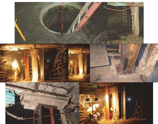
Entrance to the Confined Space. Span 34, Spalled Support Column with Exposed Main Rebars and Broken Stirrups. (Condition Credit: NYSDOT) Repairing the Flagged Conditions.
