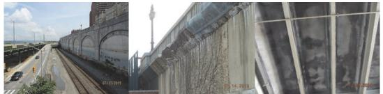
2015: Spans 19-21, East Fascia Overhang, Looking Southwest - Large Edge Spalls with Numerous Cracks and Heavy Efflorescence Throughout Overhang. Span 52 Looking South - General View of Underside of Deck Showing Extensive Dampness and Cracks with Efflorescence.
