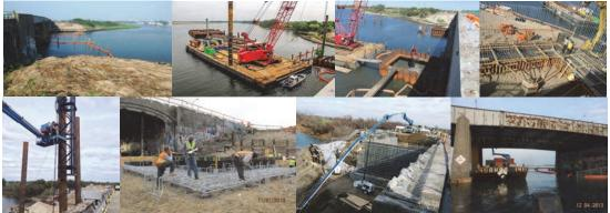
June 2013: North Side of Gerritsen Bridge - Turbidity Curtains Placed on Both Sides of Navigable Channel. July 2013: Work Barges Driving Steel Sheeting for Pier #1 Cofferdam. September 2013. October 2013: Rebars and Form Work for Footing and Walls at the Northwest Abutment. Stage 1 Piles. November 2013: Inspecting Rebar. December 2013: Tremie Concrete Pour at Pier #2. Inspecting Spans 7 and 8 of the Existing Bridge From a Barge. (Inspection Credit: NYSDOT)
