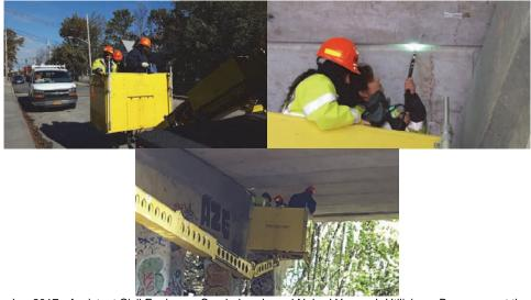
November 2017: Assistant Civil Engineers Sarah Jurado and Nahed Yaaqoub Utilizing a Borescope at the Van Name Avenue Bridge Over B&O Railroad (Abandoned) in Staten Island. The Snooper was Operated by Assistant City Highway Repairer Derrick Butler.
