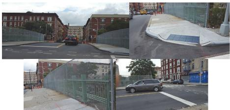
East 187<sup>th</sup> Street Bridge over Metro North After Construction – Asphalt Overlay. Southwest Pedestrian Crosswalk. New Chainlink Fence. North View.
