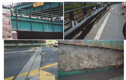
South and North Fascia - Along the Fascias are Built-Up Riveted Steel Girders. The Steel Railing Posts are Welded at the Base to the Top Flange of the Fascia Steel Girders. Deterioration of Joint at Abutment. Underside of Deck with Scaling and Efflorescence.
