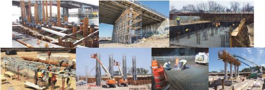
Mill Basin January 2016: New Pier #9. Cofferdam With 24-Inch Steel Shell Pipe Piles. Existing Moveable Span at Upper Right. March 2016: Scaffolding in Place at Pier #11 for Flag Repairs of Existing Bridge. North Abutment at Right.
