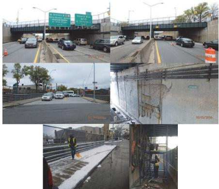
49<sup>th</sup> Street Bridge Over Grand Central Parkway. May 2016: Elevation Left and Right. Beginning Approach. Begin Abutment at Bays 9 to 14 - Spalls With Exposed Corroded and Debonded Rebars and Hollow-Sounding Concrete Areas. (Credit: NYSDOT) December 2017: Snow Removal. Erecting Scaffolding at the Abutment.
