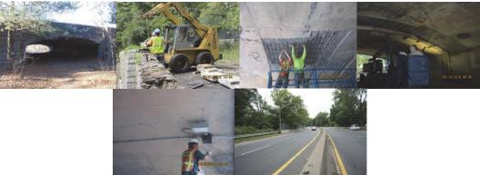
Mosholu Parkway Bridge over Equestrian Path. (Credit: NYSDOT) Bridge Before, During (Removing Stones and Stone Masonry, Removal and Repair of Deteriorated and Unsound Concrete, Repairing the Underdeck Lighting), and After Construction.
