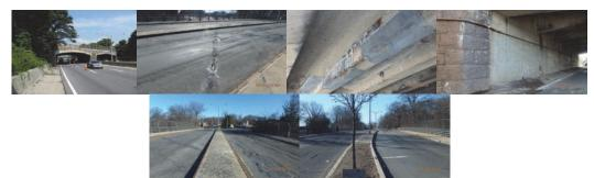
Douglaston Parkway Bridge Northbound Over Cross Island Parkway. March 2016: Top of Bridge, Asphalt Wearing Surface Above Beginning Abutment - Spalls and Uneven Wearing Surface. Span 1 - Deteriorated Concrete Covered With Wire Mesh. Abutment End. Approach Begin and End. (Credit: NYSDOT)
