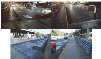
January 2017: Bridge Grating. October 2017: Span 9, Right Side, Eastbound Travel Lanes. The Top of the Steel Open Grid Deck has Multiple Steel Plates Installed Throughout the Eastbound Lanes to Cover the Damaged Areas of the Gratings. Span 9 Right Sidewalk. (Credit: NYSDOT)
