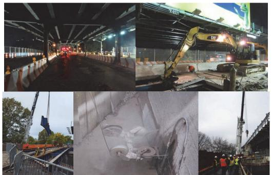
Night Work in August 2017. Stage 1 Deck Demolition in September. Stage 1 Steel Demolition Girder Removal in November 2017. December 2017 - Stage 1C Wire Saw Cutting at The West Abutment. Lifting Out the Cut Pieces.
