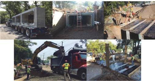
Midland Avenue Culvert in September 2017 – Precast Sections. Looking East - Precast Box Culvert Section Installation Complete. Looking North – Completed Installation of Waterproofing Membrane on the Outside of all Joints. Excavating. Assistant Civil Engineer Tatyana Krushelnitskaya (on Left) Inspecting the Waterproofing of the Culvert Box.
