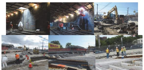
January 2017: Shielding Installation Below the Bridge Deck and Above the Railroad Tracks. Debris Removal Through Protective Shielding. February 2017: Stage 1 Demolition of Pavement and Concrete Overlays. March and May 2017: Stage 1 Demolition of Concrete Bridge Deck and Beam Encasements. May 2017: Site Visit – Assistant Civil Engineer Daniel Smith, Deputy Commissioner Robert Collyer, Community Liaison Nancy Catapano, and Resident Engineer Joe Catapano.
