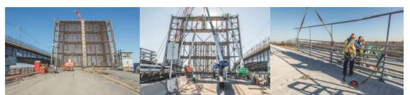
December 2017: South Leaf of the Mill Basin Bridge During Demolition. Sidewalk and Median Removed. The New Bridge is at Left Carrying Eastbound and Westbound Belt Parkway Traffic. North Leaf of the Mill Basin Bridge During Demolition. Steel Bridge Deck, Median, and Walkways are Removed. New Mill Basin Bridge is at the Right Side. Erecting the 7-rail Bridge Rail and Fence at the East Side of the Bridge for the Bicycle/Pedestrian Walkway.
