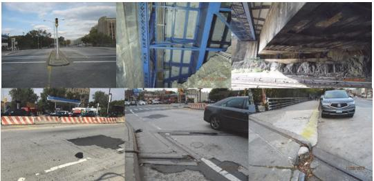
Top of Bridge. June 2016: Roadway Deck Underside of Span 1, Transverse Cracks With Efflorescence and Hollow Sections. (Credit: NYSDOT) September 2016: Southeast Portion of the South Abutment - Underside Framing. September 2017: Jersey Barriers on Beginning Approach. November 2017: Beginning Abutment Joint Northbound Roadway (Right Side) - Depressed Sealant, Missing Armor and Concrete Header. Left Curb Adjacent to Beginning Joint - Missing Steel Face. (November Credit: NYSDOT)
