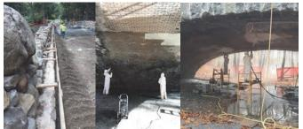
October 2016: Concrete Curb Layout. November 2016: Cleaning the Bricks Under the Bridge Arch. December 2016: Cleaning the Historic Stone Masonry and Removing Graffiti.
