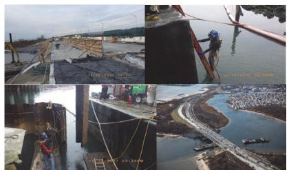
December 2017: Wood Forms Erected on the Bridge for the Future Concrete Barrier Separating the Pedestrian/Bicycle Walkway from the Future Eastbound Belt Parkway Traffic. Pedestrian Fence Anchor Bolts at Left. Diver at Pier # 2 Entering the Waterway to Cut the Steel Cofferdam Sheeting Prior to Removal. Removing Steel Sheeting Cut from Cofferdam #2. Gerritsen Inlet Bridge in December 2017.
