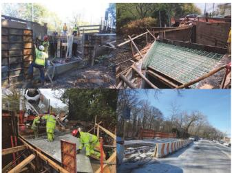
October 2017 – West Walls and Wingwalls Formwork. Looking West - Formwork and Rebar for the Roof Slab. Placing Concrete for the Roof Slab. Sidewalk.
