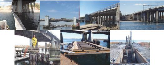
October 2015: Temporary Walkway on North Side of Bridge for Access to Pier #9. Elevation Left Span Elevation Right Span 8, 9-14, 1-7. (Inspection Credit: NYSDOT) November 2015: Extracting Wood Piles From the Existing Bridge Fender System at New Pier #9 Site. Pier #9 Steel Framing for the Cofferdam on the West Side of the Existing Bridge. December 2015: Outfall #2. Pressure Treated Wood Piles – Facing East.
