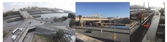
Fender System Rehabilitation Began in Summer 2017. Aerial View Prior to Construction. General View of the Fender and the Swing Span. Removal of the Existing Timber Rubbing Strips From the Fender.
