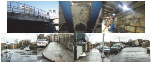
East 162<sup>nd</sup> Street Bridge over Metro North Before Construction. May 2016: Span 1, Underside of Deck Exhibits Longitudinal Cracks With Efflorescence. End Abutment Stem. (Credit: NYSDOT) Northeast Side. Southwest Pedestrian Crossing. North Sidewalk. East View.
