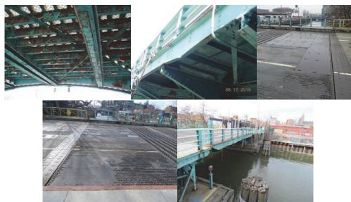
Union Street Bridge - 2016: Severe Corrosion and Peeling Off Paint Under Deck of Span #3. Span 3 -The Left Fascia Stringer Exhibits Impact Damage. (Impact Credit: NYSDOT) April 2017: Steel Plates Covering the Steel Grid Deck. December 2017.
