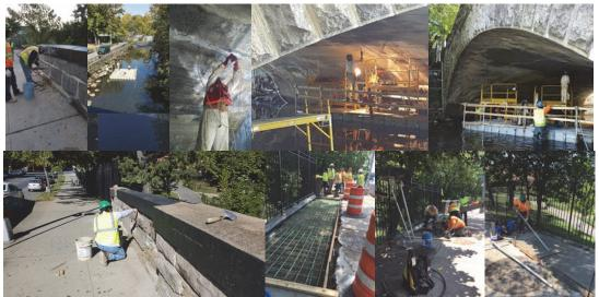
East 180<sup>th</sup> Street Bridge During Construction – South Parapet Wall, Working Platform, Crack Repairs, and Tuck Pointing. Sidewalk Repairs.
