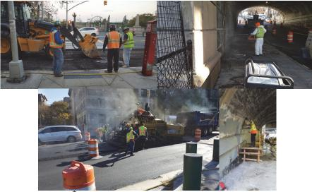
Riverside Drive Bridge over West 138<sup>th</sup> Street During Construction – Asphalt Milling, Power Washing, Asphalt Placement, and Weep Hole Drilling.
