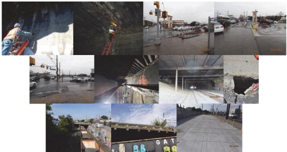
2010 Inspection - Hands-On Inspection of a Pier. Obtaining a Steel Coupon Sample From a Stringer. March 2015: Looking West, South, and East Across Bridge Deck. April 2015. October 2015: Elevation Right. Span 2 Right Parapet - The Outer Face Exhibits Spalls With Exposed Rebars. Spans 1 and 2 New Right Side Sidewalk. (Credit: NYSDOT)
