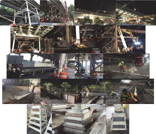
Steel Repairs at the Viaduct Began in Summer 2017. Temporary Supports for New Strut Replacement. Temporary Shoring Tower System Assembly. "Flying" 12T Jacking Beams from Top of Viaduct and "Sliding" Them Below the Viaduct Atop the Supports. Removing Existing Column. Installing New Column. Sawcutting and Removing the Deck. Removing Existing Floorbeam. Steel Roadway Plates Placed Over the Cut Section of the Deck. New Floorbeam Installation. New Column Wheelguard.
