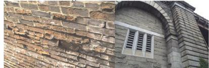
Brooklyn Approach Arch Block I: Deteriorated Brick on the East Face of the Barrel Wall. South Elevation - Staining and Loss of Mortar at the Joints and Arch Stones.
