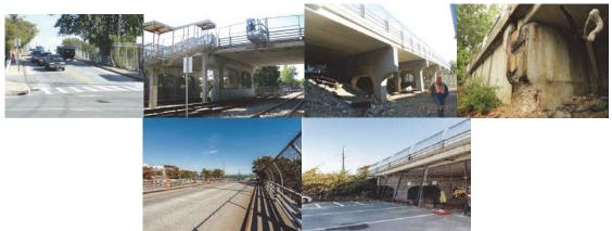
Hannah Street Bridge Over SIRT South Shore. Spans 1-4 - Right Elevation. October 2015: Large Deep Spall on Right Corner of Beginning Abutment. (Credit: NYSDOT) Before Construction.
