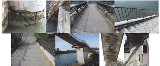
Bridge Conditions in June 2014. Pier 1 Over the East River – Close-up of 2 Wide Cracks. Begin Abutment Stem Right Side - Failing Patch and Map Cracking. Span 1 Deck Wearing Surface. Span 2 Railing. Span 3 Concrete Steps. Pier 2, Under Span 2, Looking Southwest – Spalled Concrete Area With Exposed Rebar at Bottom of Pier. Underdeck of Span 1. Begin Abutment Stem.
