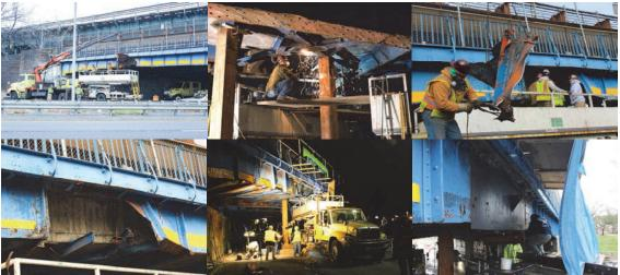
On January 9, 2016, a Truck Travelling South on the Parkway Struck the Bridge, Causing Damage to a Fascia Girder and its Preceding Girders, Stringers, and the Hanging Bars of a Strongback. Crews Responded, Cut a Portion of the Sheared Girder and Spliced it With a New Section and Installed Shoring.
