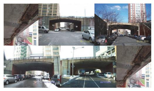
In general, the arch bridges have an adequate load-carrying capacity, however, there are areas of map cracking and visible leakage through the joints. Mesh has been installed at the underside of the deck to prevent debris from falling on vehicles or pedestrians below.
