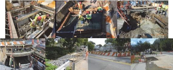
August 2017 - Looking Northwest - Constructing Falsework to Support the Culvert Roof Slab. Pouring Concrete for the Stage 2 Roof Slab. Contractor Excavated and Demolished the Existing Culvert for the Final Stage Along the South Side of Forest Avenue. September 2017 - Concrete Placement at Culvert Walls. Construction of Culvert Opening. Temporary Barrier. Looking West - Contractor Placed Concrete for the Sidewalk, and Seed and Topsoil at Unpaved Areas.
