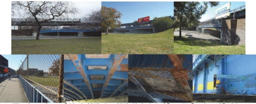
Westchester Avenue Bridge in 2015. June 2016: Underdeck of Span #1 - Deteriorated Deck is Shielded With Timber Planks and Wire Mesh. Bent Stiffener at Span #1.
