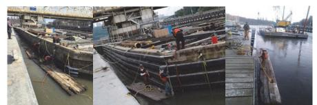
Installation of New Lumber on the Existing Fender. Building an Extension at the Northeast Side of the North Fender with New Lumber.
