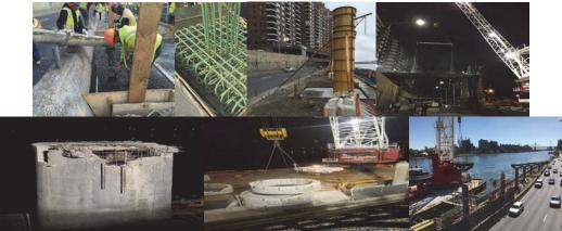
Installing Rebar Cages and Pouring Concrete for Pile Caps. Installing Pier Caps and Removing the Old Bridge. Demolishing the Concrete Tower. Installing the Hub and Arms. (Credit: NYCDDC)
