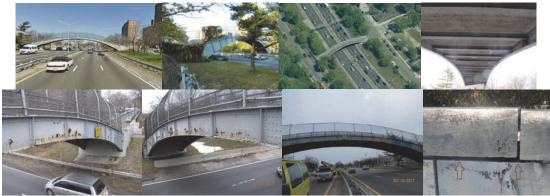
27<sup>th</sup> Avenue Bridge – Existing Conditions. March 2016 - Underside of Deck has Several Areas of Spalling Concrete With Wire Mesh Shielding. February 2017. Missing Mortar on Beginning Approach Wall in September 2017.
