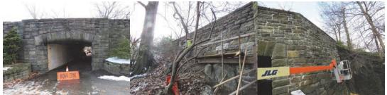
December 2017: Maintenance Workers Adding Mortar to the Joints on the Beginning and Ending Right Side Wing Walls of the Margaret Corbin Drive Bridge over Pedestrian Path Near the North Entrance.
