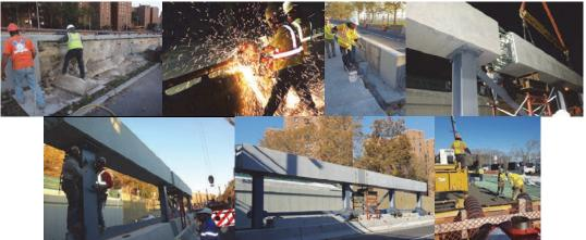
October 2016. November 2016: Stage 2 - Final Bolting and Alignment of Precast Pier Cap Segment. December 2016: Placing and Finishing Concrete for Deck Slab.
