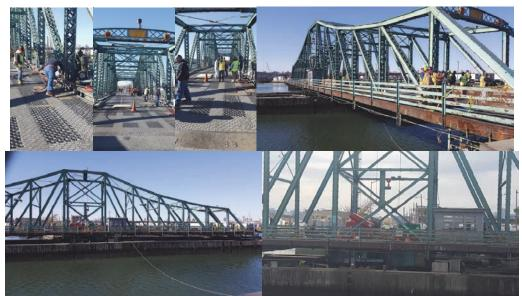
November 2017: Division Crews Addressed Multiple Red PIA Flags on the Grand Street Bridge. Work Included the Repair, Replacement, and Reinforcement of Stringers on Spans #1 and #2 as Well as Repairs to the Deck Grating and Roadway Plates. (Credit: Earlene Powell)
