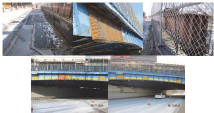
2016: Span 1 Right Sidewalk Near Beginning Abutment – Steel Plates. Girder Reinforced With New Steel Plate and Angles. Strongback Girder at Right Side of Span 1. Right and Left Fascia. (Credit: NYSDOT)
