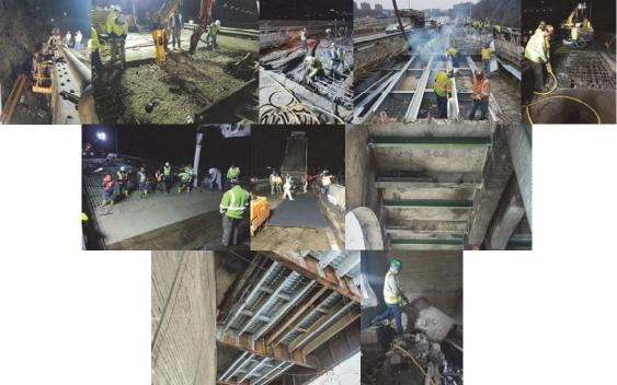
March 2017. Deck Removal During Northbound Repairs. Concrete Placement for Full-Depth Deck. Asphalt Placement Over Cured Deck. April 2017: Newly Installed Steel Angles Under Span 38, and Steel Installed Above the Harlem River Drive.
