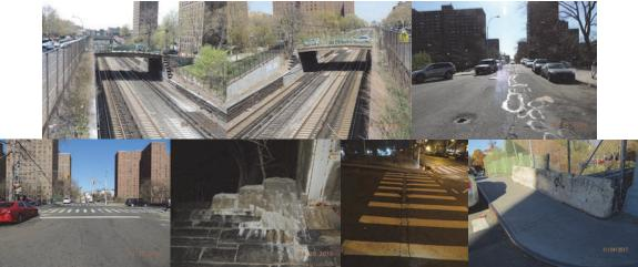
East 169<sup>th</sup> Street Bridge: April 2016 - Left and Right Elevations. Beginning and End Approaches. Moderate Map Cracking With Efflorescence in the Reinforced Concrete at the Top of the Beginning Right Wingwall. (Credit: NYSDOT) February 2017: End Abutment, Joint with Deck. Full Length Cracks With Deteriorated Wearing Surface. November 2017: Left Sidewalk Near End Abutment - Temporary Jersey Barrier in Place.
