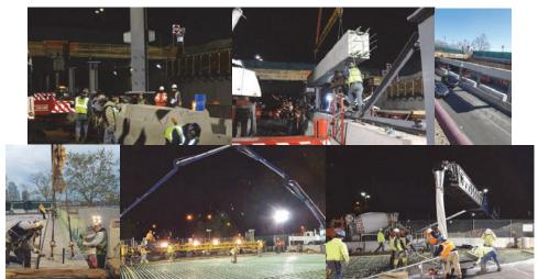
April 2017: Stage 3 - Erection of New Steel Columns and Pier Caps at the Center Pier. Alignment of Final Hollow Slab Unit for Stage 3. May 2017: Concrete Placement for Stage 3 Bridge Deck. June 2017: Concrete Placement for South Sidewalk and Median.
