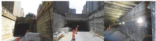
July 2017: Elevation South and North. South Portal Segment, Looking Northeast - Concrete Slab on Grade is Removed. Temporary Lighting Fixture Installed on the East Liner.
