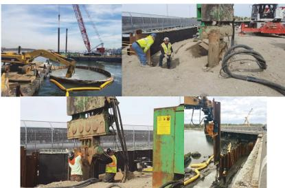
April 2017. May 2017: Removing Steel Sheeting From the East Approach. The Sheeting was Utilized to Create a Protective Cofferdam in the Area. A Wall of Steel Sheeting was Also Installed Ahead of the Reconstruction of the Esplanade.
