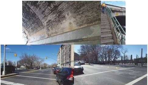
Riverside Drive Bridge over West 138<sup>th</sup> Street After Construction – Weep Holes Installed, Railing Painted. New Asphalt Overlay – North and South Views.
