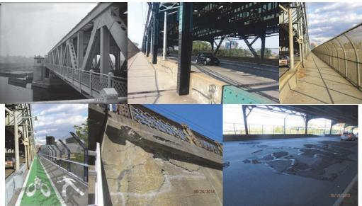
Roosevelt Avenue Bridge – In 1927. (Credit: NYC Records). Looking East. Existing and Proposed Bicycle/Pedestrian Path. 2014: Right Wingwall at the End Abutment. The Top Exhibits an area of Diagonal Cracks With Efflorescence and Spalls. The Deteriorated Concrete Areas are in Safe and Stable Condition. 2015: Spans 26and 27 – Examples of Uneven Asphalt Patches and Broken Concrete Areas. (Credit: NYSDOT)
