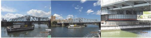
Madison Avenue Bridge in 2016: Left and Right Elevations Spans 12 to 15. Pier 13 – Existing Rack and Pinions. (Credit: NYSDOT)
