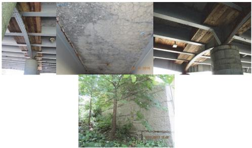
June 2015: Span 1 Deck – Hollow Sounding Concrete Areas are Covered by Timber Planks That are in Good Condition. April 2016: Span 2, Underside of Deck, Bay 3 - Exhibits Scaling, Mapcracking with Localized Efflorescence, and Dampness Over Approximately 50%-60% of its Surface. (Credit: NYSDOT) July 2016: Span 2 Timber Shielding. July 2017: Cladding on the Left Side of the End Abutment in Good Condition.
