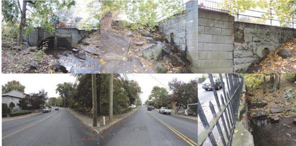
Forest Avenue Bridge Over Clove Lakes Park Stream. November 2017: Right Elevation at Upstream. Beginning Abutment Right Wingwall. End Abutment Stone Masonry Wingwall. Beginning and End Approaches. Right Side Parapet and Concrete Coping. (Credit: NYSDOT)
