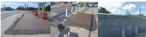
August 2016: Span 2 Left Sidewalk Looking South - Location of the Through Hole. Span 1 Right Sidewalk Looking North. Spalled and Cracked Areas on Top of Span 2 Parapet. (Parapet Credit: NYSDOT)
