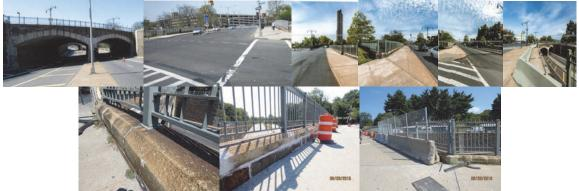
Southern Boulevard Bridge over East Fordham Road Before Construction. West Side, East Side, Eastbound Roadway, and Missing Section of Fence. August 2016: Cracked Cap Stone at Right Wingwall. Repaired Joints on Right Parapet. Jersey Barriers and Fence Above the Deck on Span 1.
