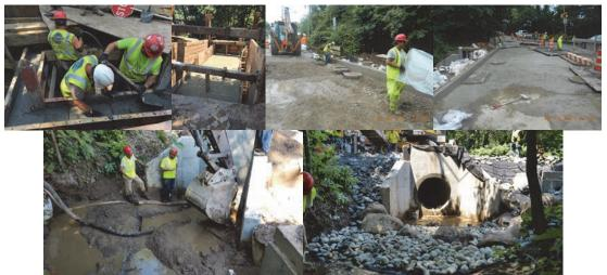
June 2017 – Pouring Manhole Walls. July 2017 – Placement of Low Strength Concrete Complete. Placement of Concrete Curb Along the South Gutter Line. Placing Roadway Base. Excavation of Material on Top and in Front of the Apron Slab. Placement of River Bed Stones, Medium Stones, and Boulders Adjacent to the Culvert Walls and Apron Slab.
