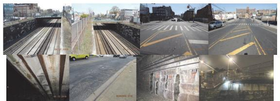
East 180<sup>th</sup> Street Bridge: April 2016 - Left and Right Elevations. Beginning and End Approaches. May 2016: Diaphragms in Bay 2 Exhibit Underside Spalling With Exposed, Debonded Rebar. (Credit: NYSDOT) September 2016: The Left Side of the Roadway Looking Toward the Beginning Abutment - The Wearing Surface Exhibits an Uneven Surface, Map Cracking and Small Potholes. February 2017: End Abutment Looking Northeast. Water Leakage Stains on the Bottom Portion of the Stem. Night View.
