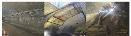
July 2017: West Tunnel Liner, Looking West - Efflorescence and Water Leakage and Missing Mortar Between the Masonry Stones. North Side End of Brick Arch, Looking Southeast - Missing Section of Metal Ceiling Liner and Mortar Between Bricks. East Side of Tunnel, Looking Northeast - Installation of New Drainage Pipe.
