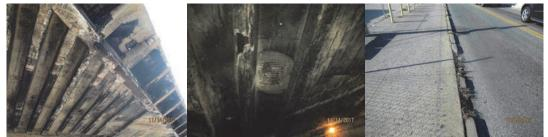
Span 2, Underside of Deck- Spalled Concrete Encasement and Deck. Exposed Rebar. Span 2, Top of Deck - Spalled and Missing Sections of Curb With Vegetation Growth. (Credit: NYSDOT)
