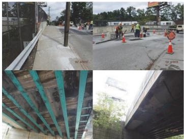
Arthur Kill Road Bridge Over SIRT South Shore. October 2016: Left Sidewalk. Repairing the Wearing Surface at the Beginning Right Side Near the Beginning Abutment. The Wearing Surface has Widespread Cracks and Uneven Asphalt Concrete Patches. Span 1 Underdeck General View of Timber and Wire Mesh Shielding. Stable Hollow-Sounding Areas and Shallow Spalls With Scaling and Efflorescence. (Credit: NYSDOT)
