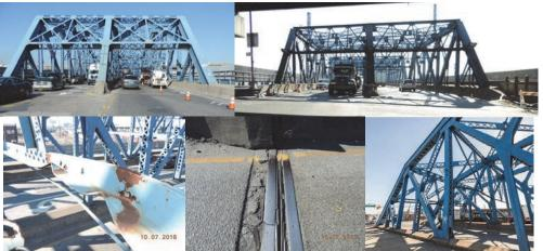
Leggett Avenue Bridge over Amtrak Before Construction. October 2016: Begin and End Approaches. Span 1, Bottom Sway Strut Bracing Exhibits Severe Deformation and Several Upward Bent Sections due to Vehicular Impact. End Abutment Transverse Deck Joint Steel Armor is Cracked. Deck Joint Header Exhibits Shallow Spalls. (Credit: NYSDOT) Southeast View.
