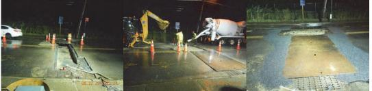
Arthur Kill Road Culvert over Ridgewood Avenue in August 2017 - Cut Back Asphalt Wearing Surface. Placing Concrete Base. Plates Installed Over Trench for the New 20 Inch Diameter Iron Pipe.
