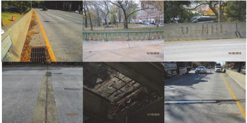
West 94<sup>th</sup> Street Viaduct – 2015: Span 34 Left Lane. Span 12 Right Railing and Left Side Concrete Parapet. Span 31 Top of Deck. 2016: Span 4 – Spall With Exposed Rebar. Pier # 3, Deck Joint, Northbound Henry Hudson Parkway, Left Lane – Joint Missing Metal Plate. (Credit: NYSDOT)
