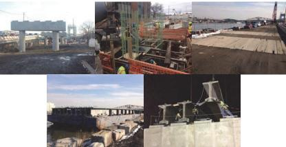
January 2017 – Mini Piles. February 2017 - Erection of the Concrete Beam – Timber Planks Over the Relieving Platform. Concrete Beams on Barge. (Credit: Artemio Angeles) Span 2.
