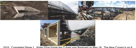
2015: Completed Stage 1. Water Flow Inside the Culvert was Restored on May 18. The New Culvert is an 8 Foot by 7 Foot Concrete Box - About a 3x Larger Capacity. April 2015: - Installation of the Pedestrian
