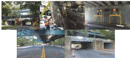
Roosevelt Avenue Bridge in July 2015: Elevation Right. (Credit: NYSDOT) Before, During (Stone Masonry Preparation, Underdeck Concrete Repair), and After Construction.
