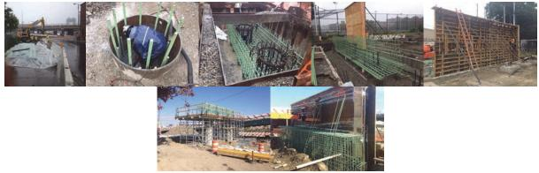
September 2016: North Abutment Pier 8 Foundation. Epoxy Reinforcement Bars to be Installed at South Abutment are Covered. Removing Concrete With a Chipping Gun. Reinforcement for Pile Cap. North Abutment -Reinforcement for the Stem and Forms. October 2016: Contractor Continued Installing Reinforcement and Forms for the North Abutment. November 2016: Pier 3 of Southbound Roadway - Pier Cap Almost Ready for Concrete Placement. November 2016: South Abutment Stem Wall. (Credit: Artemio Angeles)
