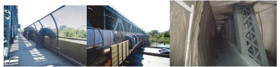
September 2016: - The Contractor Employs a Vacuum System to Capture Lead Particles During the Lead-Abatement Process. This is Done Using Negative Air Pressure to Prevent Emissions From the Abrasive Blasting Process Used to Remove Lead Paint. All Blasting is Done Within Negative Air Containment Units to Protect the Public From Emissions. View Inside the Containment – Bascule Span, Looking East.
