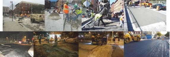
East 187<sup>th</sup> Street Bridge over Metro North During Construction – July and October 2016. Top of Span 1 – Wearing Surface Paved With New Asphalt. Deck Repair. Installing Waterproofing. Asphalt Placement.
