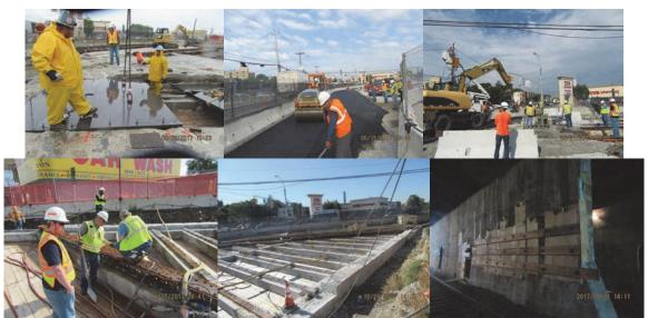
May 2017: Installing 2" Thick Steel Plates to Prepare for a Temporary Road Surface, Under Observation by Assistant
