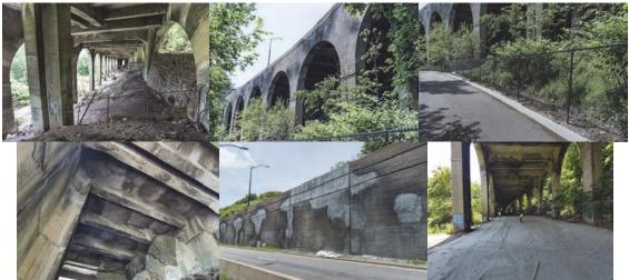
May 2017: Spans 36 to 25. Shotcrete Arch Repairs on Spans 34-32. Fence Restoration. Shotcrete Deck Repairs. Rebuilt Parapet.
