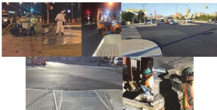
East 165<sup>th</sup> Street Bridge Under Construction. Summer 2016. Asphalt Placement. New Pedestrian Ramp. Bridge Jacking. Bearing Replacement.
