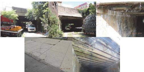
Southern Boulevard Bridge Over CSX. July 2016: Elevation Left and Right. Begin Abutment Stem Exhibits Vertical and Horizontal Cracks With Efflorescence, and Isolated Areas of Hollow-Sounding Concrete. Left Sidewalk at End Abutment. (Credit: NYSDOT) September 2016: Right Side Under Deck of span #1 – Mold is Present and the Bottom Flanges are Corroded.
