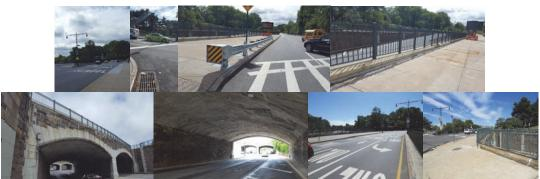
Southern Boulevard Bridge After Construction - New Asphalt at West Side and at the Eastbound Roadway. New Guiderail and Fence. Section of Fence. Repaired Joints at Fascia. Sealed Crack and Installed Weep Holes at Westbound Fordham Road. September 2017: Barriers Removed After Construction – Top of Span 2 Looking East. Top of Deck at Beginning Approach Looking West.
