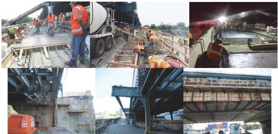
June 2017: West Viaduct – Stage 1 Placing the Sidewalk. August 2017: East Approach – Stage 1 – Placing Sidewalk Concrete. October 2017: West Viaduct – Stage 1 Filling the New Roadway Grid Deck With Concrete. Span 22. Span 20, Left Side, Impact Damage Location. (Spans 20 and 22 Credit: NYSDOT)
