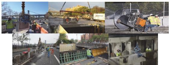
April 2016: Demolition of West Barrier Wall at Exit Ramp. May 2016: Saw Cutting the Existing Deck. Saw Cutting and Demolition of West Barrier Wall at Entrance Ramp. Erecting Forms for West Barrier Wall at Exit Ramp. July 2016: Saw Cutting and Demolition at West Abutment Wall.
