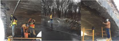
January 2017: Tuck Pointing the Bricks. Power Washing the North Parapet Wall. February 2017: Underdeck Brick Removal - the Extent of the Deteriorated Bricks was Not Known Until Multiple Layers of Existing Paint Were Removed From the Underside Surface of the Bridge Arch.
