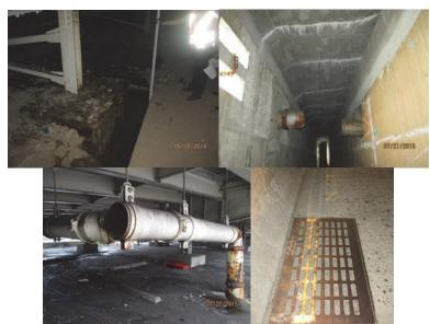
Scour Hole at Pier #3 in 2014. 2015: Span 5 – Right side. Span 46 – Left Side. Downspout Near North Abutment. (Credit: NYSDOT) Typical Clogged Scupper Inlet.
