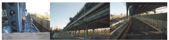
October 2016: Installing the New North Sidewalk – West Viaduct, Looking East. November 2016: Contractor Demolishes the Sidewalk over Van Wyck Expressway. East Viaduct – Stage 1 Installing the North Sidewalk Steel. December 2016: Installed North Sidewalk Stringers. West Viaduct – Roadway Deck Removed.
