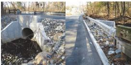
November 2017 – Half of the Culvert is Rehabilitated – Beginning and Ending Approach Right Side Embankments are Repaired. New Guide Railing, Bridge Railing, Curb and New Asphalt Pavement.
