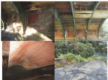
Pier 1 Solid Stem Wall Between Bays 4 and 5 – the Lower Portion of the Pier End Face (Below the Timber Shielding) Exhibits Efflorescence, Dampness and Leakage Over a Large Area. Span 2, Underside General View. Span 2, Underside Brick Arch at Girder Near Pier 2 Exhibits Efflorescence over Most of the Surface Area. Span 3, Left Parapet and Railing Interior Face. (Credit: NYSDOT)
