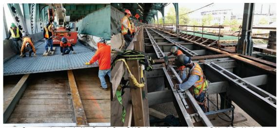
Contractors Installing the New Bascule Span Grid Deck on the Roosevelt Avenue Bridge in Flushing in March 2017. The Bridge is Permanently Set in a Closed Position Since the Late 1950's. Installing Haunch Angles at the West Viaduct Roadway Deck in July 2017.
