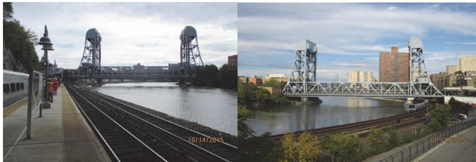
Broadway Bridge – West and East Elevations.
