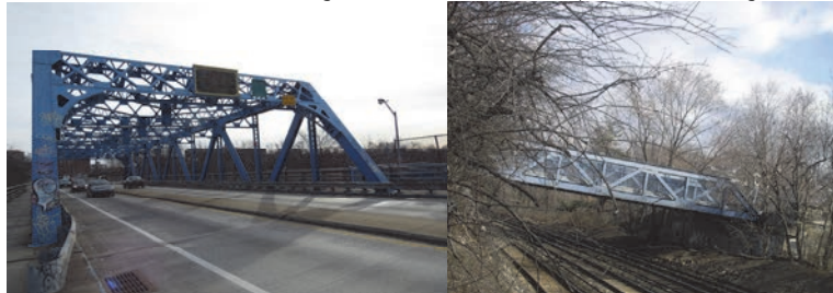
East 174 th Street Truss Bridge over Sheridan Expressway and 204 th Street Pedestrian Bridge over Metro North in 2017.
