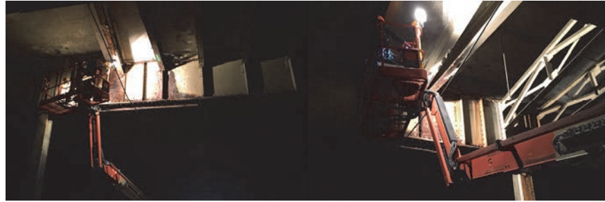
Field Measuring for Steel Repairs in September 2017.
