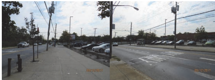
September 2017 – Right Sidewalk and Roadway Wearing Surface.
