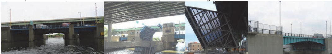
Unionport and Hamilton Avenue Bridge. (Open Credits: NYSDOT) Union Street Bridge. Greenpoint Avenue Bridge. (Greenpoint Credit: Michele N. Vulcan)
