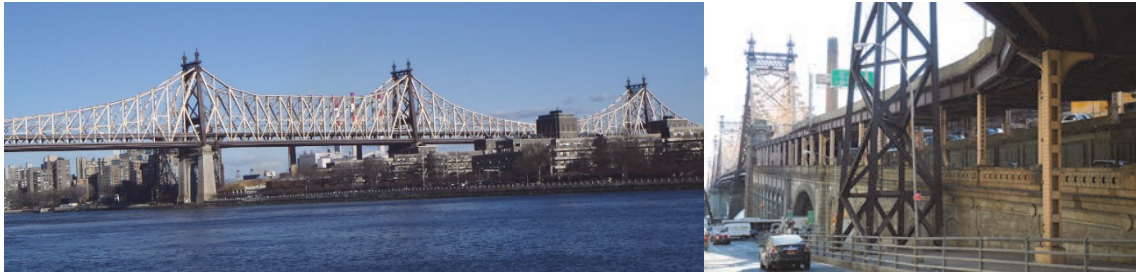
Ed Koch – Queensboro Bridge. (Credit: NYSDOT)
