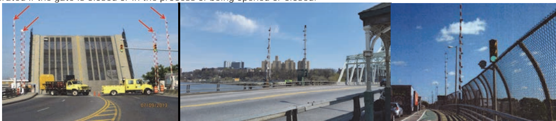
Metropolitan Avenue Bridge over English Kills Warning Gates. (Credit: NYSDOT) West 207th Street/West Fordham Road Bridge Warning Gate. Greenpoint Avenue Bridge over Newtown Creek Southwest Warning Gate.
