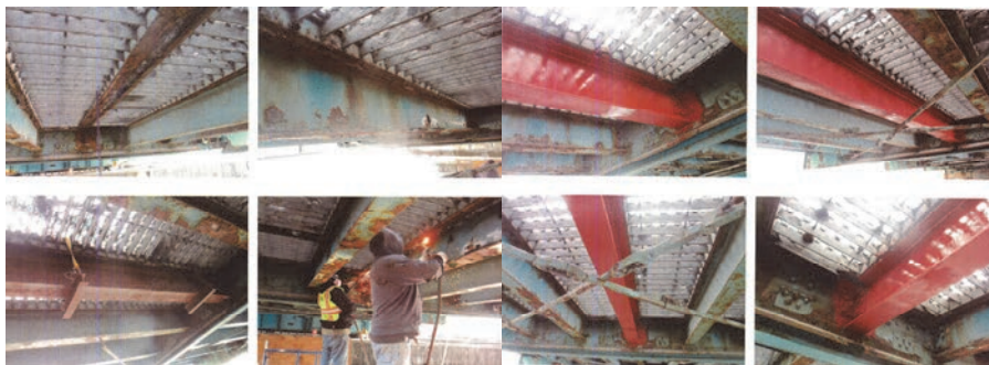
December 2016: Removing and Replacing a Severely Corroded Stringer Under Span 1 on the Grand Street Bridge over the Newtown Creek.
