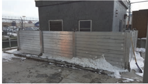
2017: Completed Ninth Street Bridge Flood Barrier.
