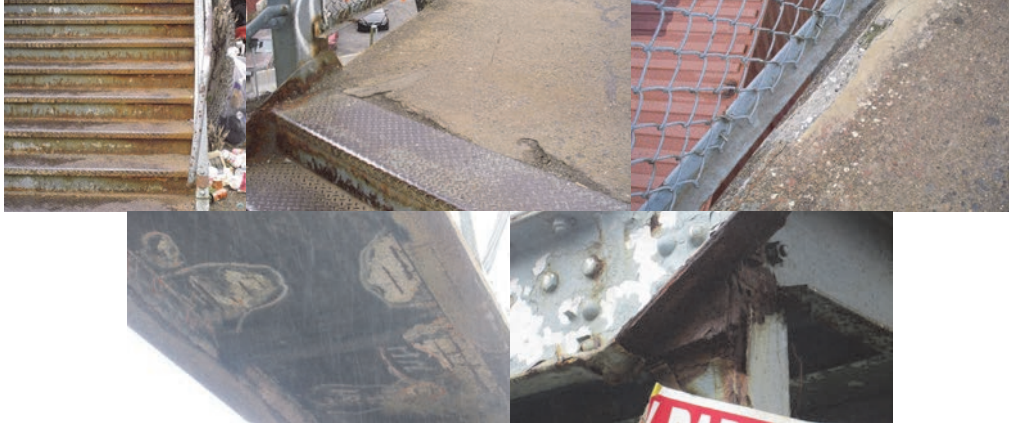
Existing Conditions: Rusted Steps and Damaged Railing. Deteriorated Deck. Spalled Concrete Deck on Main Span. Spalled Concrete – Underside of Deck. Deteriorated Steel.
