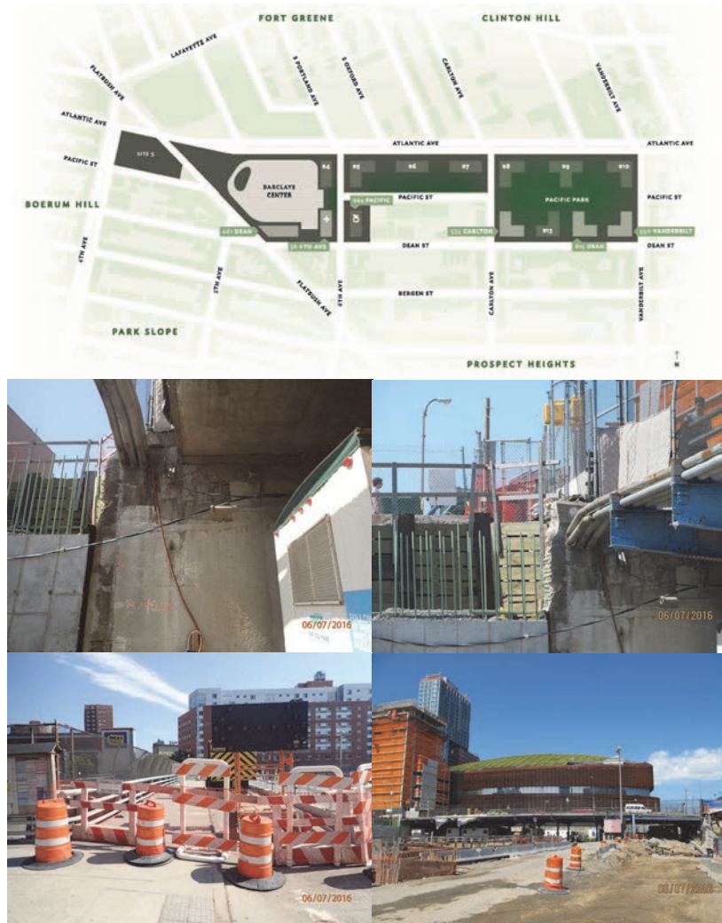
Pacific Park Site Map. (Credit: Greenland Forest City Partners) 6/7/16 6 th Avenue Bridge over LIRR Atlantic Avenue. Begin Abutment Right Edge and Right Wingwall – a Large Part of the Wingwall was Saw Cut and Removed During the Ongoing Pacific Park Project. Beginning Approach - Left Sidewalk is Closed due to Ongoing Construction Next to the Bridge. Right Elevation. (Credit: NYSDOT)
