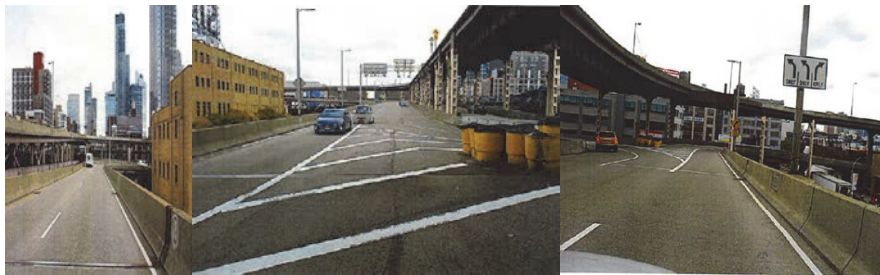
Ramp to 21 st Street After Construction.
