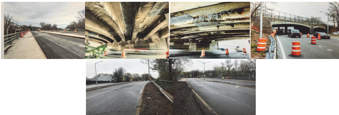
Douglaston Parkway Bridges Before Construction.
