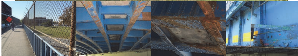
Westchester Avenue Bridge in 2015. June 2016: Underdeck of Span #1 - Deteriorated Deck is Shielded With Timber Planks and Wire Mesh. Bent Stiffener at Span #1.
