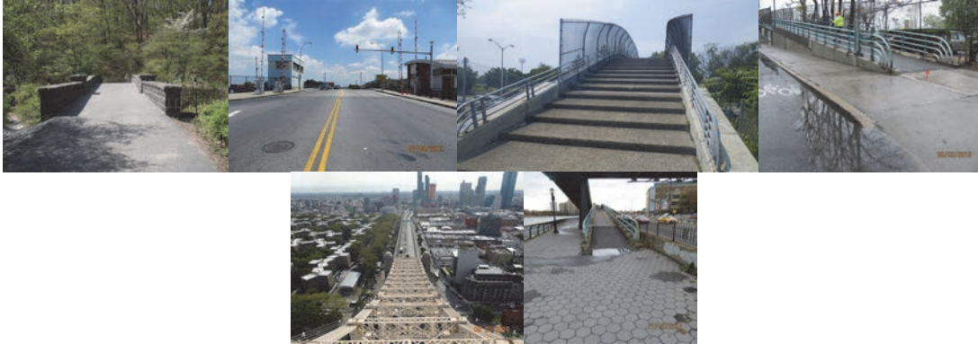
End Approach to Bridge Over Dam at Clove Lake. Metropolitan Avenue Bridge Approach. (Metropolitan Credit: NYSDOT) Belt Parkway Bridge over 26 th Avenue Approach. (Credit: Artemio Angeles) Begin Approach to Delancey Street Pedestrian Bridge Over FDR Drive. Ed Koch - Queensboro Bridge Approach. End Approach to East 120 th Pedestrian Bridge Over FDR Drive. (QBB and East 120 th Street Credit: NYSDOT)
