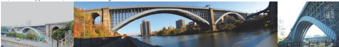
Washington Bridge. (Credit: NYSDOT) Washington Bridge in 2008. (Credit: Duane Bailey-Castro) 2010.
