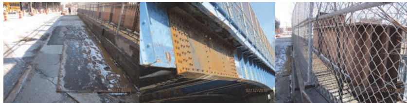
Westchester Avenue Bridge in 2015. June 2016: Underdeck of Span #1 - Deteriorated Deck is Shielded With Timber Planks and Wire Mesh. Bent Stiffener at Span #1.
