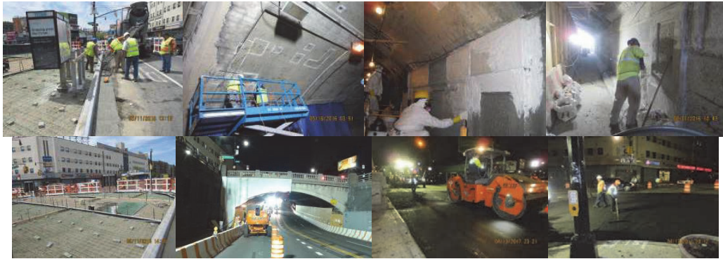
East Fordham Bridge During Construction.
