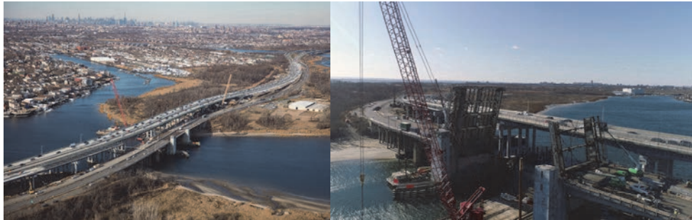
Mill Basin Bridge in December 2017.
