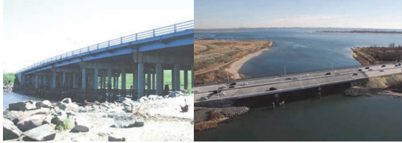
Old Fresh Creek Bridge. New Bridge in November 2013. (2002 Credit: NYSDOT)
