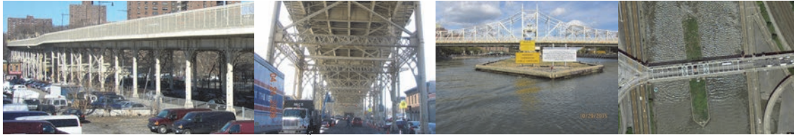
West 155 th Street Viaduct. The Timber Fender.
