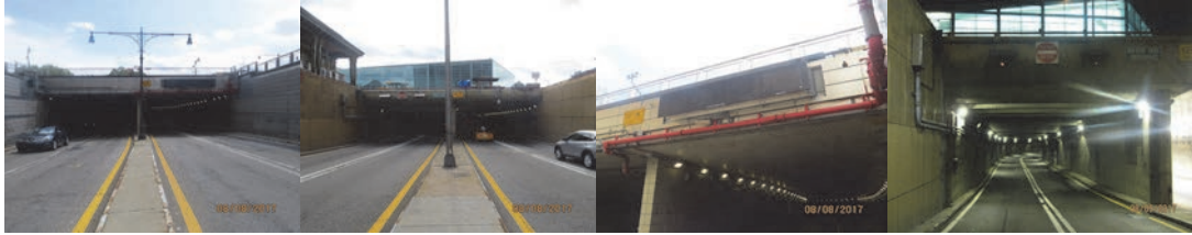
August 2017: Battery Park Underpass Elevation South and North. South Tube North Portal. Variable Message Board Will Be Replaced.
