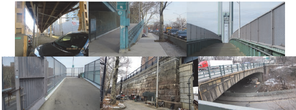
Winter 2017: Thomson Avenue Ramp of Ed Koch – Queensboro Bridge, Wards Island Pedestrian Bridge. 145 th Street Bridge. West 181 st Street Bridge over Ramp to Washington Bridge.
