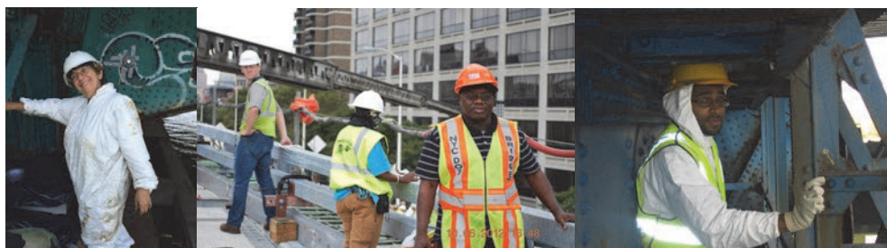
Assistant Mechanical Engineer Vera Ovetskaya on Union Street Bridge During a Strain Gauge Test. On the Bridge to her Right is an Electronic Inclinometer That Records the Angle of the Bridge Opening. Brooklyn Bridge Engineer-in-Charge Ohene Duodu. Engineering Technician Christopher Brathwaite Assisting in Strain Gauge Balance Testing on Unionport Bridge in October 2010.
