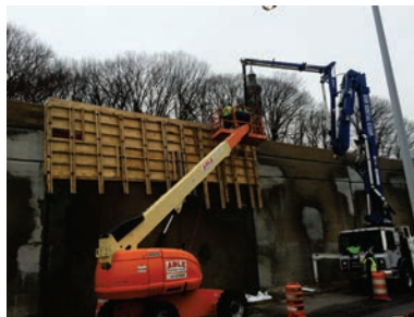
Trans-Manhattan Connector Ramp Under Construction in January 2017.
