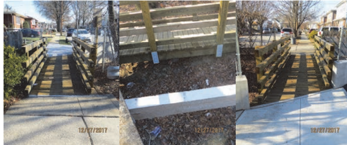
Galloway Avenue Culvert in December 2017.
