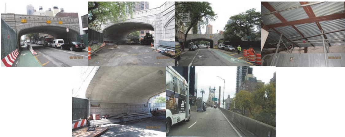
Ramp to the Ed Koch – Queensboro Bridge from East 58 th Street over East 59 th Street Before Construction. June 2016: Westbound Span 11 Vertical Clearance Signs. Span 10 – Left Elevation. Spans 10 and 11 – Left and Right Elevations. Span 8, Underside of Deck at Bay 2. Steel. Stay-in-Place forms Installed as Shielding. Pier 11. (Credit: NYSDOT)
