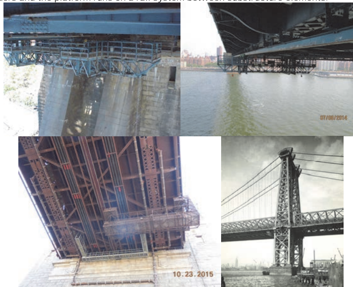
Manhattan Bridge and Ed Koch - Queensboro Bridge Travelers. (Credit: NYSDOT) Williamsburg Bridge in 1942: First Traveler in Place at the Brooklyn Tower. Second Traveler Shown on Scow Prior to Lifting.
