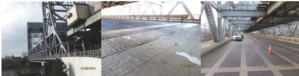
2015: Framing Span 2. November 2016: Pier 1, Finger Joint at Southbound Roadway - Misaligned Fingers. December 2016: Span 2, Northbound Roadway - General View of Steel Grid Deck. (Credit: NYSDOT)
