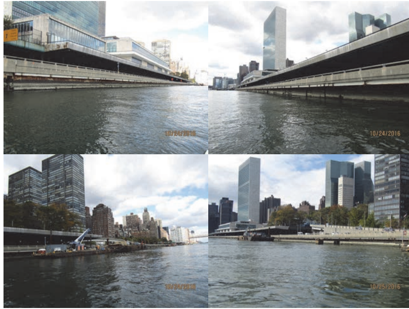
October 2016: Right Elevations. (Credit: NYSDOT)
