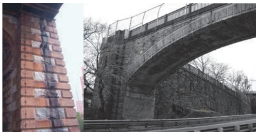
East Face of Brooklyn Bridge North Stem Wall. (Credit: NYSDOT) West 176 th Street Pedestrian Bridge Beginning Abutment Stem Wall.
