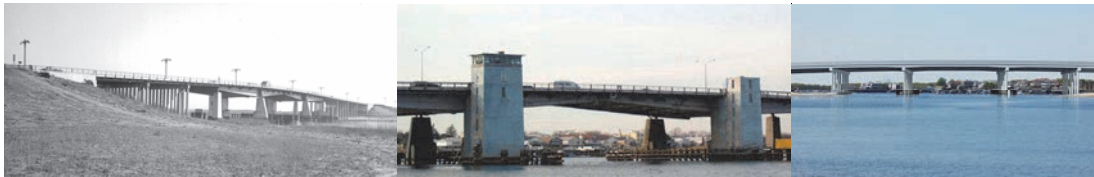
Mill Basin Bridge in 1946. Old and Proposed Bridge.
