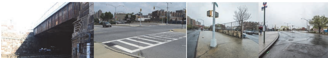
East 165 th Street Bridge Over Metro North Before Construction.
