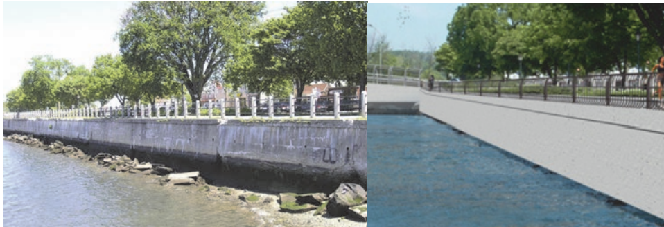
Existing Seawall. Proposed Treatment.
