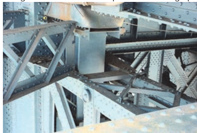
Truss Bearing on Manhattan Bridge. (Credit: NYSDOT)
