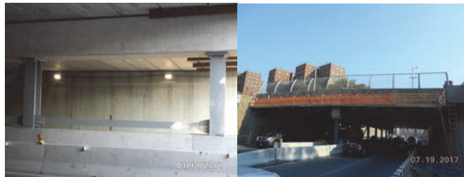
July 2017: Pier 1 New Columns of the Main Bridge. Elevation Right. (Credit: NYSDOT)
