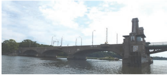
July 2017: Left Elevations Spans 4 – 7. (Credit: NYSDOT)
