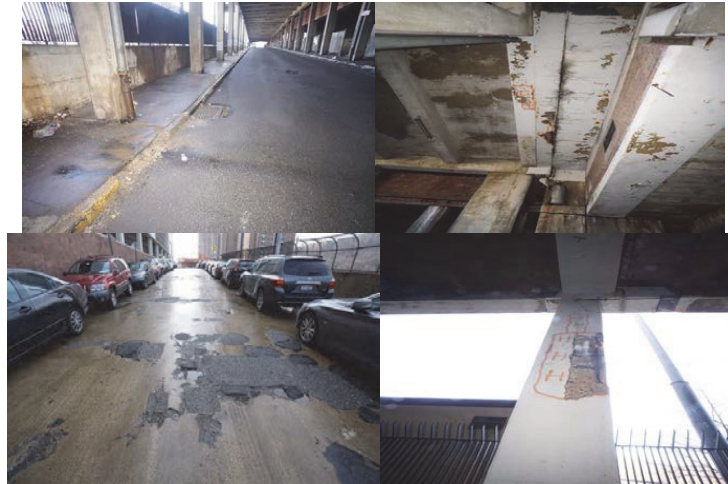
Matthewson Road Bridge over MacCracken Avenue Before Construction.
