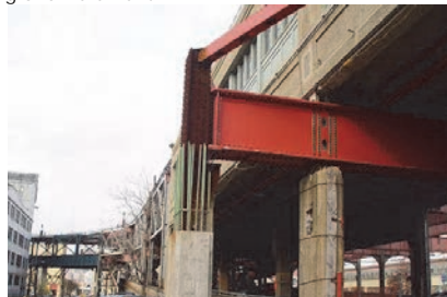
Ed Koch Queensboro Bridge Bent Column Ready for Jacking in 2005.
