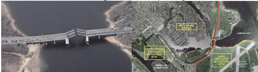
Old Open Bridge. Freshwater and Tidal Wetland Mitigation Sites.
