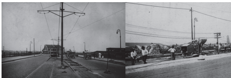
Traffic on the 145 th Street Bridge in 1921, and Roadway Repair in 1922.
