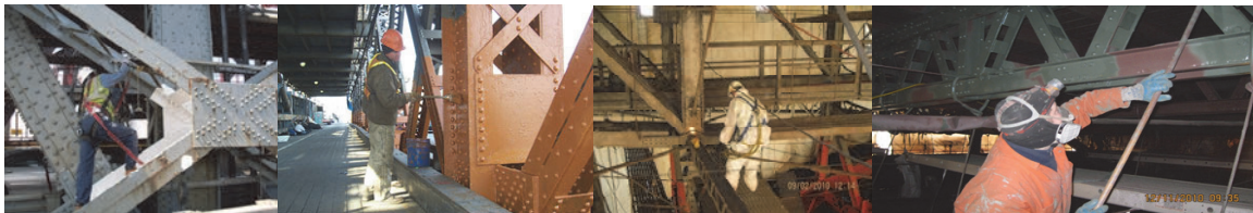
Williamsburg Bridge in June 2010: Application of Finish Coat at North Truss Diagonal. Salt Splash Painting on the Williamsburg Bridge. (Salt Splash Credit: Fouad Althaibani). Inspection of Blasting Surfaces Inside the Franklin Square Arch Containment in September 2010. Brooklyn Bridge Main Span Painting in December 2010.
