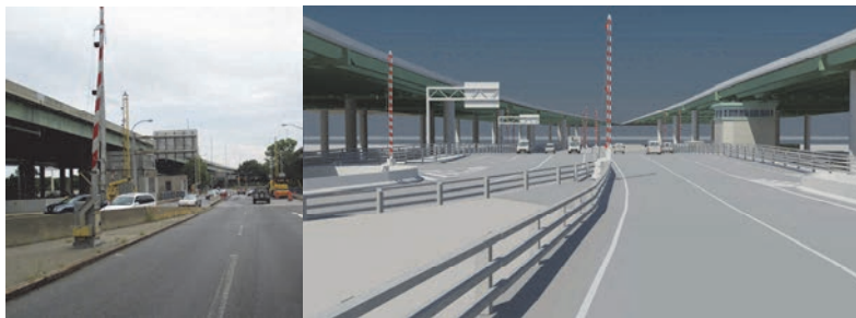
Looking East – Towards Current And Proposed Bridge.
