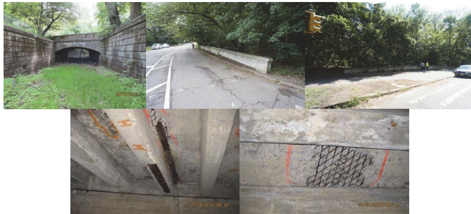
East Drive Bridge over Bridle Path Before Construction.
