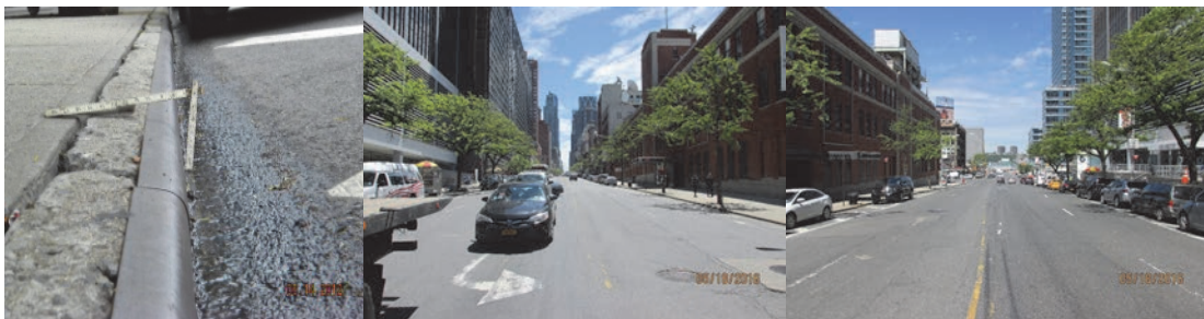
West 57 th Street Bridge over Amtrak. 2016: Beginning and Ending Approaches. (2016 Credit: NYSDOT)
