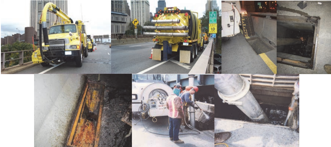
Drain Truck on Brooklyn Bridge Ramp. (Credit: Peter Basich) Drain Cleaning on the Williamsburg Bridge in September 2011. (Credit: Shaikh Islam) Cleaning Catch Basins on the Manhattan Bridge.
