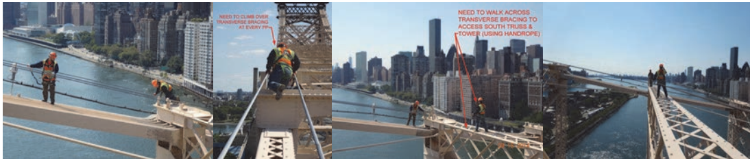
Inspecting the Ed Koch – Queensboro Bridge. (Credit: NYSDOT)
