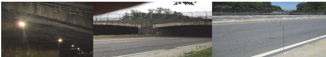
Douglaston Parkway Bridges After Construction.
