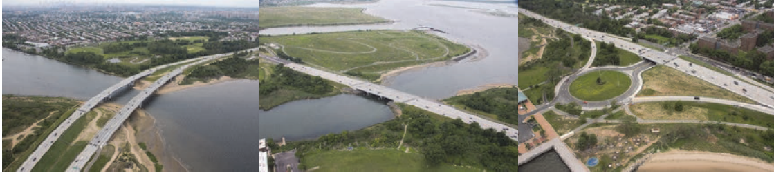
Summer 2014: Paerdegat, Fresh Creek, and Rockaway Parkway Bridges.
