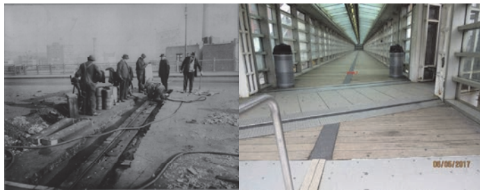
Constructing an Expansion Joint on the Riverside Drive Viaduct in 1918. Joint for Span 7 on the Chambers Street Pedestrian Bridge in 2017.
