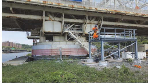
2016: Macombs Dam Bridge CO2 Containment.
