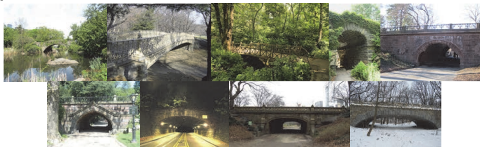
East 62 nd Street Pedestrian Bridge (Gapstow Bridge) over the Pond. West 62 nd Pedestrian Bridge (Pinebank Arch). West 77 th Street Pedestrian Bridge (Ladies Pond Bridge) in 2016. Central Park West Drive over the Loch Stream from the Pool (Glen Span Arch) in 2017. (Ladies Pond and Glen Span Credit: Eugene Parker) East Drive (Trefoil Arch) in 2017. (Credit: Michele N. Vulcan) Greywacke Arch (East Drive Bridge Opposite East 80 th Street) in 2011. East Drive Bridge over Transverse Road #3 in 2015. West Drive (Dalehead Arch) in 2016. Highland Park Pedestrian Bridge.
