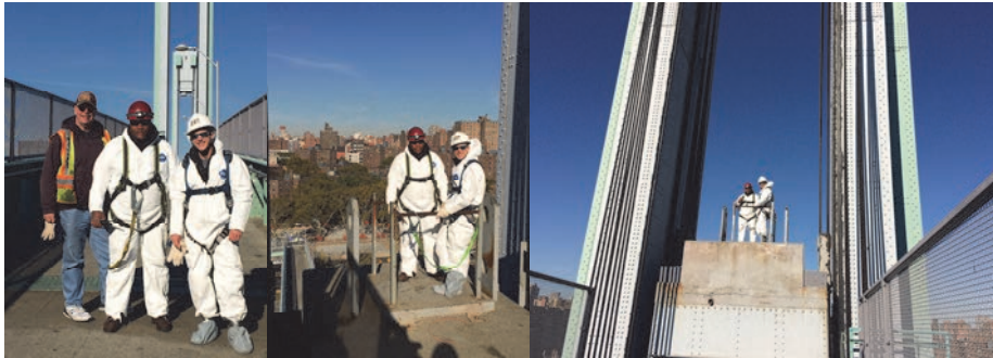
October 2017: Maintenance Crew Riding on the Wards Island Pedestrian Bridge Counterweight to Reach the Top of the Tower and the Machinery Room. Oilers Steven Marxhausen and Rene Francis and Assistant Mechanical Engineer Nazariy Davydovych. Oiler Rene Francis and Assistant Mechanical Engineer Nazariy Davydovych on the Bridge Counterweight and Secured to the Railing. Counterweight Rising.
