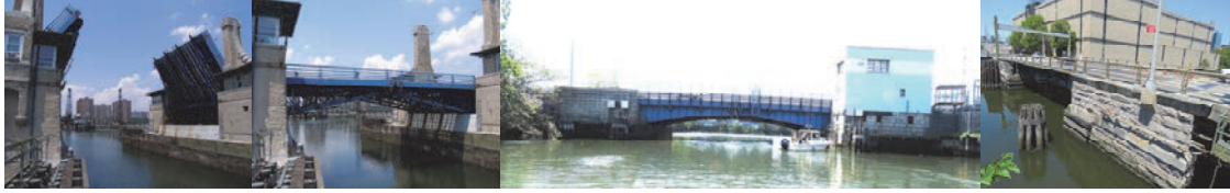
Shore Road Bridge in July 2011. (Credit: Sergey Parayev) Metropolitan and Hunters Point Avenue Bridges.
