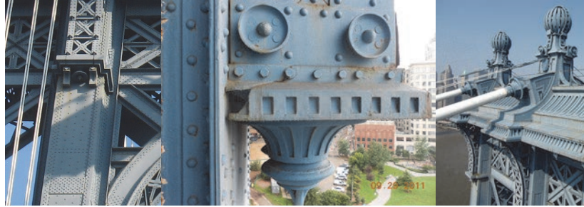
Ornamental Bordure, Horizontal Plate Supporting Rosette, Rosette, and Bracket. Ball, Ornamental Cable Band, Ornamental Top Castings, Rosettes and Castings, Rosettes and Ornamental Ceiling Brackets, and Bands Around the Ball.
