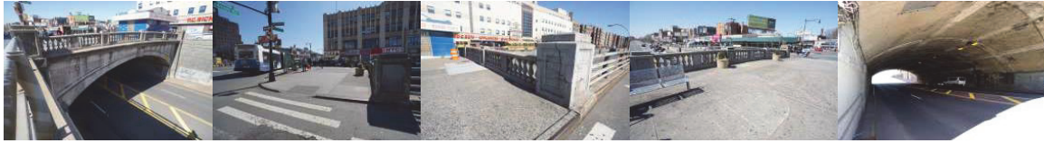
East Fordham Bridge Before Construction.
