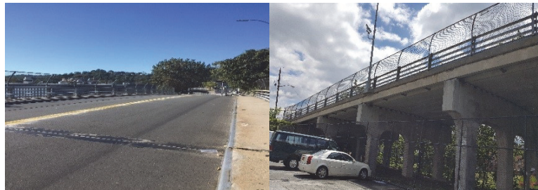
Hannah Street Bridge After Construction.
