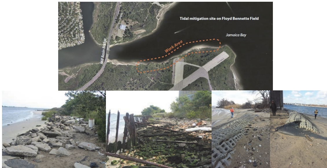
Tidal Wetland Mitigation Site. Before Mitigation – Large and Heavy Surface Debris and Deteriorated Bulkhead. Inspecting the Hurricane Sandy Damage at the Site in January 2013.
