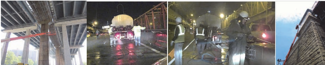
Washing the Williamsburg Bridge in July 2011 and May 2015.
