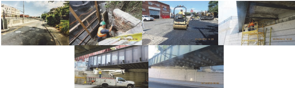
71 st Avenue Bridge over Cooper Avenue. Before, During, and After Construction.
