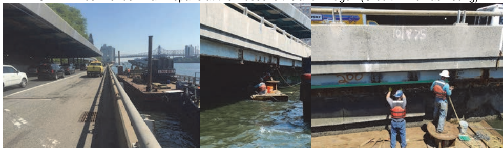
2017: Steel Repairs at the FDR Drive Cantilever Structure. (Credit: Thomas Leung)
