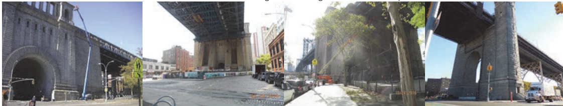
Inspecting the Exterior of the Manhattan Bridge Anchorage. Manhattan Bridge Brooklyn and Manhattan Anchorages. Ed Koch - Queensboro Bridge Queens Anchorage (Credit: NYSDOT)
