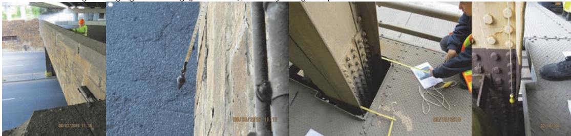
Plumb Bob in Use at Elliot Avenue Bridge over Queens Boulevard in 2016, and the Lower Level of the Ed Koch - Queensboro Bridge in 2018.
