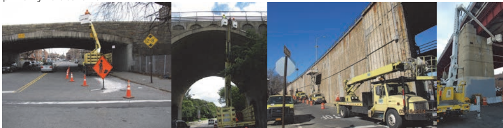
Inspecting the Belt Parkway Bridge over 26th Avenue in December 2012. (Credit: Artemio Angeles) Nereid Avenue Bridge over Bronx River Parkway in June 2012 - Using a 60 Foot Boom With Outriggers. (Credit: Bojidar Yanev) Brooklyn-Queens Expressway (Eastbound) over Cadman Plaza/Brooklyn-Queens Expressway (Westbound). Pulaski Bridge in July 2017. (Credit: Mitul Patel)
