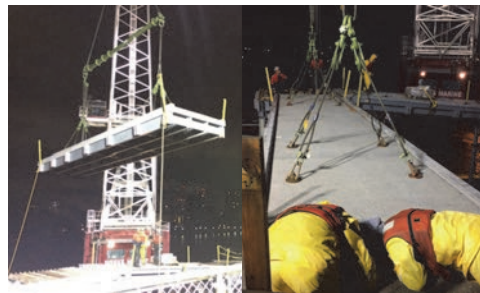
Installing the New Spans and Bridge. (Credit: NYCDDC)
