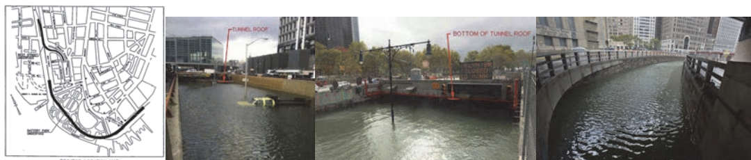
Battery Park and West Street Underpasses. October 2012 - Battery Park Underpass - View Looking West at the South Portal Entrance Near the FDR Drive. View Looking South at the North Portal Entrance Near West Street. West Street Underpass – Approach at South Portal Looking Southeast. Both Tunnels Were Flooded to Their Roofs, Which Means That all Tunnel Ventilation, Electrical, and Mechanical Systems Were Entirely Submerged in Saltwater.
