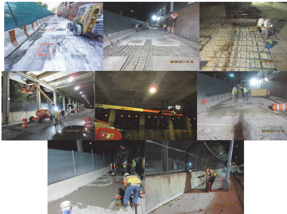
Matthewson Road Bridge During Construction.
