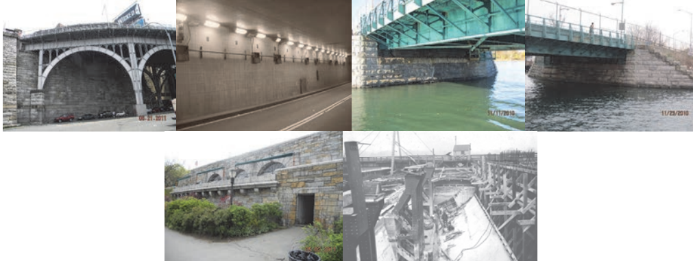
Riverside Drive Viaduct Abutment End. Battery Place Underpass Abutments. City Island Bridge Beginning and Ending Abutment. 79th Street Traffic Circle Abutment End. (Credit: NYSDOT) Constructing the Abutment of the Eastchester Bridge in 1921.
