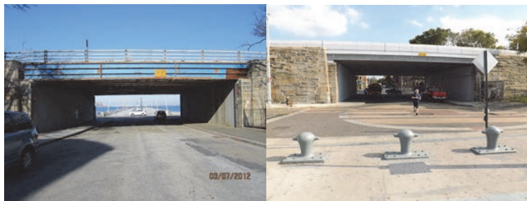
Old Bay Ridge Avenue Bridge in 2012. (Credit: NYSDOT) New Bridge in October 2016.
