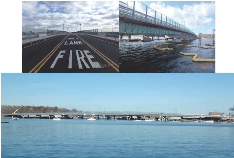
November 2017: Approach Beginning, Elevation Left and Right. (Credit: NYSDOT)
