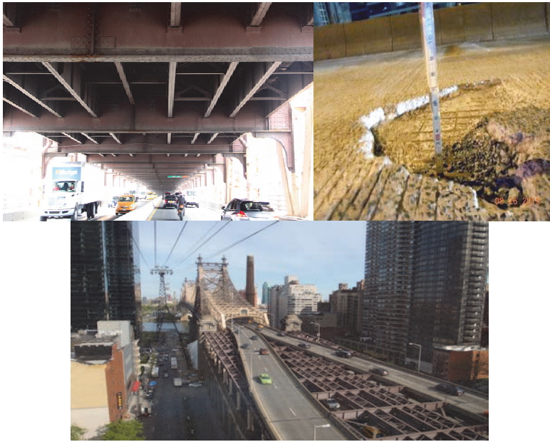
Current Roadway Condition.
