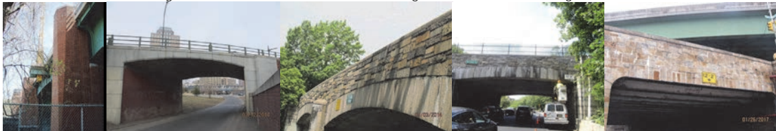
Hutchinson River Parkway Bridge. Brooklyn-Queens Expressway Over Ramp to Brooklyn-Queens Expressway (Eastbound). Right Side Fascia on the Bronx Pelham Parkway Bridge. Inspecting the Cladding Stones of the Fascia of Span 1 on West 252 nd Street Bridge Over Henry Hudson Parkway. Eliot Avenue Bridge Over Queens Boulevard.
