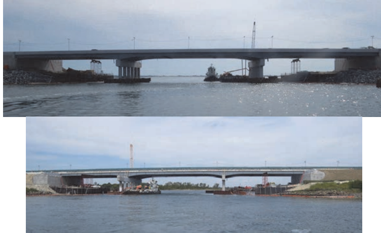
Gerritsen Inlet September 2017: Left and Right Elevations. (Credit: NYSDOT)
