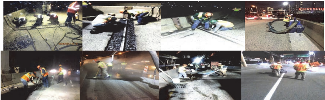
Ramp to 21 st Street During Construction.
