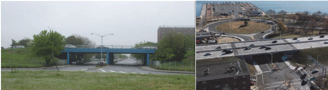
Old Rockaway Parkway Bridge. New Bridge in November 2013. (2002 Credit: NYSDOT)
