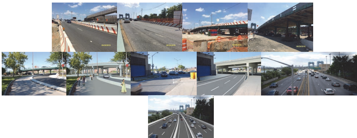
June 2016: Approach Begin and End. Left Elevation. Right Elevation Spans 3 – 7. (Credit: NYSDOT) Looking East at the 127 th Street Off-Ramp: Current and Proposed View. Looking East at 2 nd Avenue: Current and Proposed View. Looking South From 3 rd Avenue Bridge: Current Harlem River Drive and 2 nd Avenue Exit and Proposed Harlem River Drive With Left Lane Exit to 2 nd Avenue.
