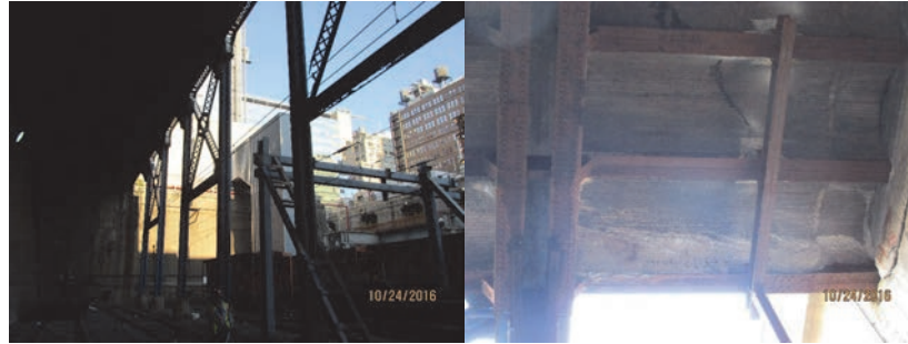
2016: Piers and 4-9. Span 1 – Underside of Deck. (Credit: NYSDOT)
