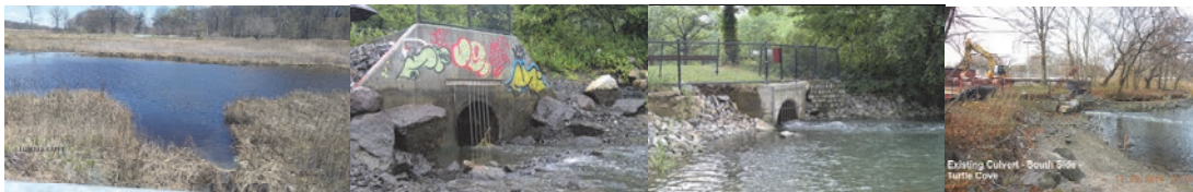
Turtle Cove. Existing Culvert – South Side.
