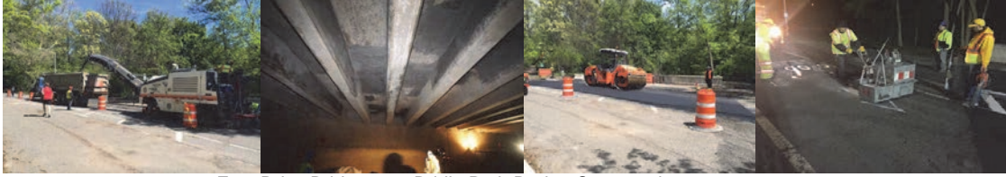
East Drive Bridge over Bridle Path During Construction.
