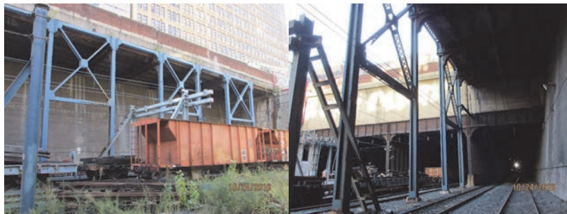
2016: Elevation Right. Piers 1-3. (Credit: NYSDOT)
