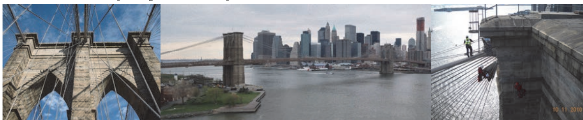
Brooklyn Bridge: 2009 Tower Closeup, 2010 View, 2010 Biennial Inspection. (2009 Credit: Emily Goodman, 2010 Credit: Jagtar Khinda, Inspection Credit: NYSDOT)
