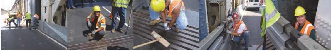
Manhattan Bridge Expansion Joint Cleaning in 2008: Supervisor Highway Repairer Thomas Cruz, Assistant City Highway Repairer Antonio Asaro, Highway Repairer Louie Dumeng, and Oiler Stanley Karolewicz. Assistant City Highway Repairers Jonathan Adorno and Antonio Asaro, Oilers Stanley Karolewicz and Ronald Grady. (Credit: Thomas Whitehouse)
