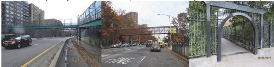
West 181 st Street, PS-5, and Carroll Street over Franklin Shuttle Pedestrian Bridges.
