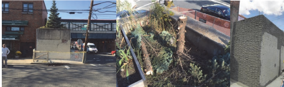
East 16 th Street Retaining Wall – Before and After Repairs.
