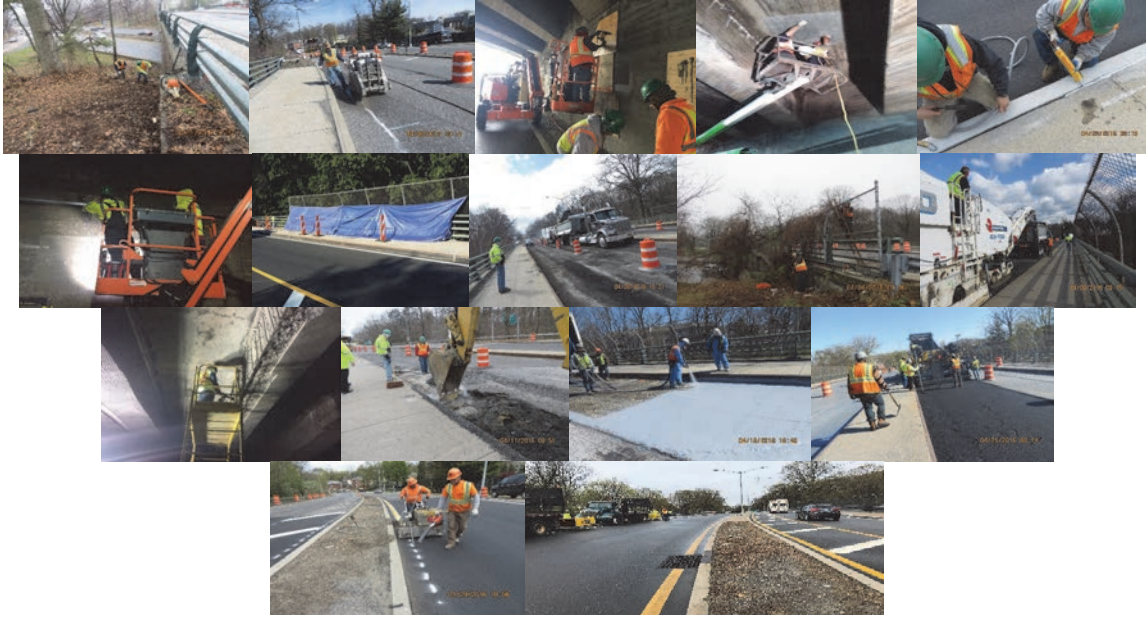
Douglaston Parkway Bridges During Construction.
