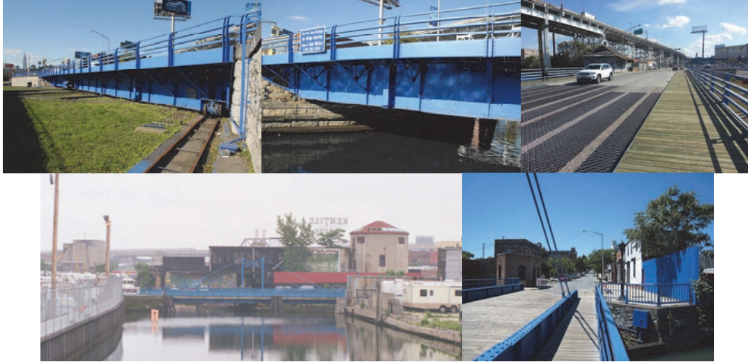
Borden Avenue Bridge. (1 st and 2 nd Credit: Peter Basich, 3 rd : Vadim Sokolovsky Carroll Street Bridge. (1 st Credit: NYSDOT, 2 nd : Russell Holcomb)
