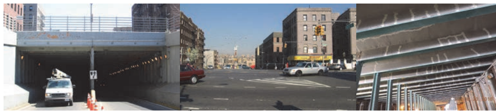
Grand Concourse Bridge over East 167 th Street. June 2016: Span 1, Repaired Underdeck and Girder Concrete Encasement. (Credit: NYSDOT)
