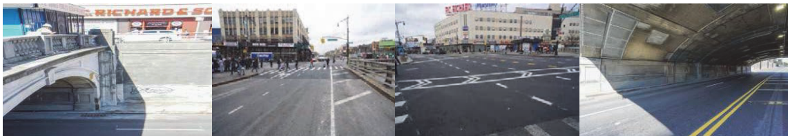
East Fordham Bridge After Construction.
