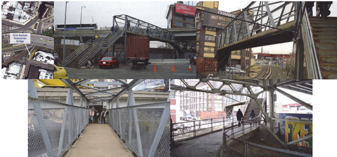
Aerial View. South Stairs and Bridge – Looking North. General View – Looking West. General View. North Stairs and Ramp – Looking South.
