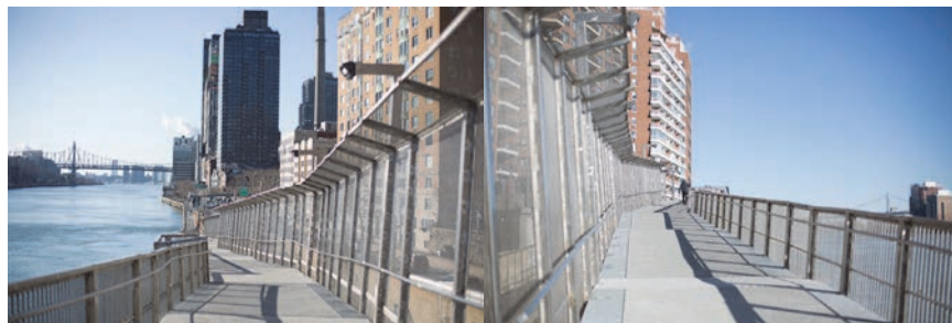
New East 81 st Street Bridge in December 2017. (Credit: NYCDDC)
