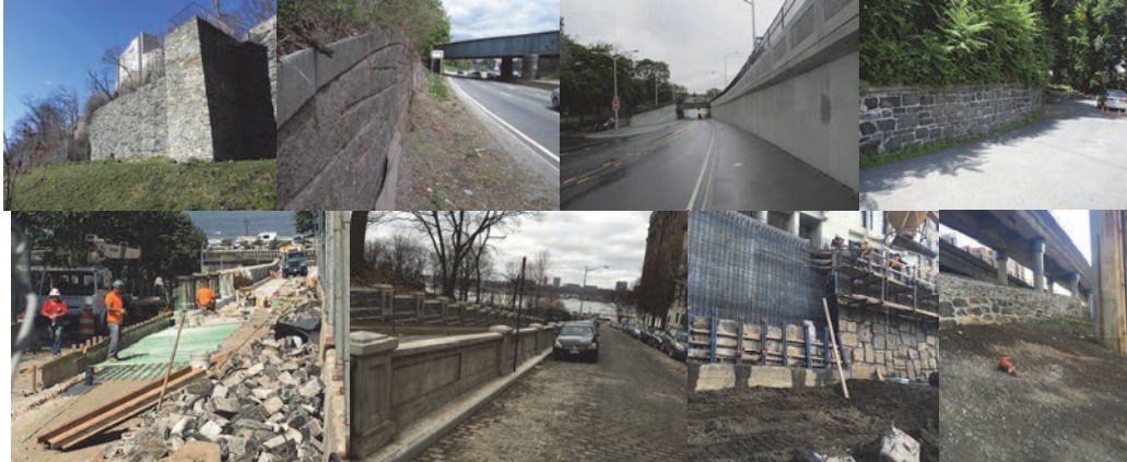
Retaining Walls: Irwin Avenue. Cross Island Parkway Southbound Before 100 th Avenue. Cooper Avenue. Douglas Road. 2016: West 155 th Street (Lower Level) Between Riverside Drive and Broadway During and After Rehabilitation by DDC. Riverside Drive (Northbound) to George Washington Bridge (West 168 th to 171 st Streets) During Rehabilitation. Riverside Drive Under George Washington Bridge Ramps (West 176 th to 177 th Streets). (2016 Credit: Jacob Ayman)
