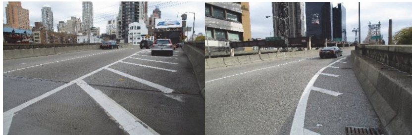
Ramp from East 58 th Street After Construction.
