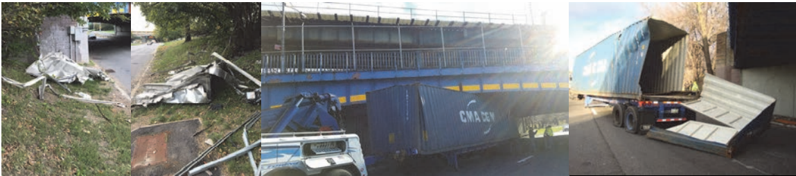
October 2016: Truck Debris Remaining at the South Side of the Bridge Along the Southbound Hutchinson River Parkway After a Bridge Strike. December 2016: Truck Tightly Wedged Under the Bridge.
