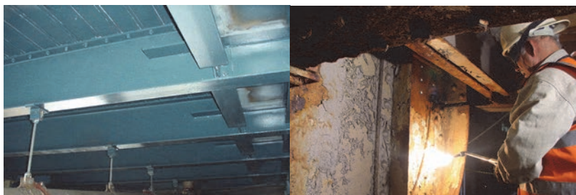
Stringers on the Manhattan Bridge. (Credit: NYSDOT) Bridge Repairer and Riveter Joseph Antony Repairing a Red-Flagged Stringer on the Bridge. (Credit: Hany Soliman)
