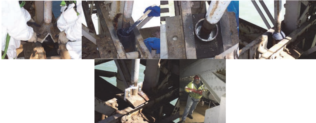
Cleaning and Lubricating the Solid Rods' Suspender Bearings on the Brooklyn Bridge. Oiler Rene Francis on the Madison Avenue Bridge During a Manual Opening of the End Lift Machinery. (Credit: Vera Ovetskaya)
