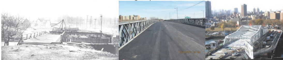
1911 Boston Road Bridge over Hutchinson River Temporary Bridge. 2011: Fresh Creek Temporary Bridge. 2004: Almost Completed New Third Avenue Span and Temporary Bridge. (Credit: Daniel Hom)
