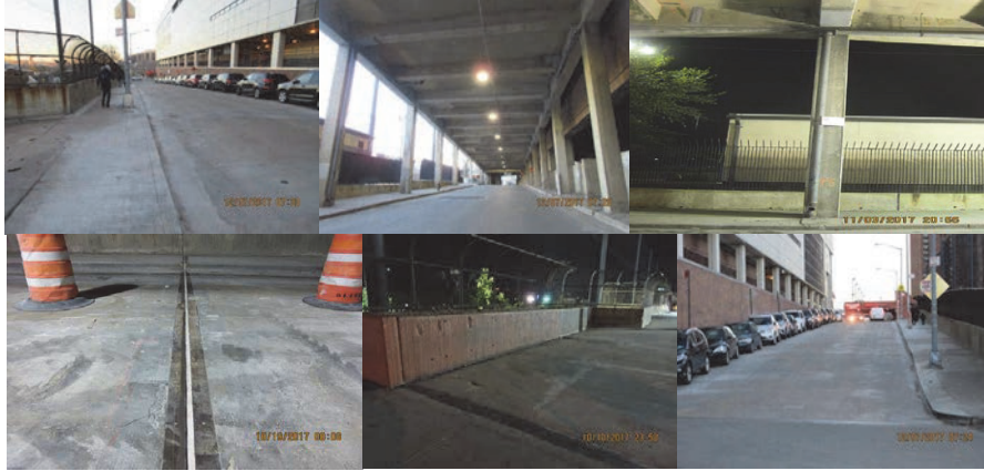
Matthewson Road Bridge After Construction.
