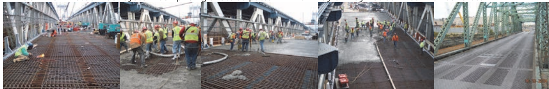
Installation of Full Width Grid Deck Panels on the Manhattan Bridge Lower Roadway in 2006. Pouring the Concrete. Grand Street Deck. (Grand Street Credit: NYSDOT)
