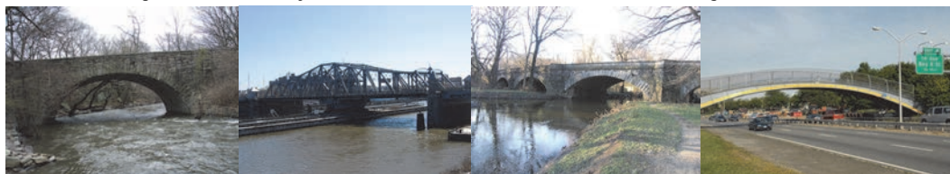
Southern Boulevard, Madison Avenue, and Mosholu Parkway Bridges. (Credit: Russell Holcomb) 17 th Avenue Pedestrian Bridge. (Credit: Peter Basich)
