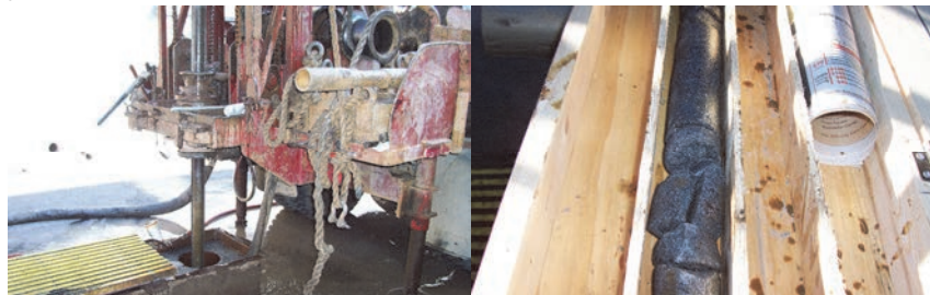
Conducting Soil Borings in 2008 as Part of the Seismic Retrofit Design of the Manhattan Bridge. Drilling to a Depth of Approximately 210 Feet to Obtain an 8-foot Long Hard Rock Sample. A 2 1/2 - Foot Long Hard Rock Sample Taken From a Depth of Between 202 and 204 1/2 Feet.
