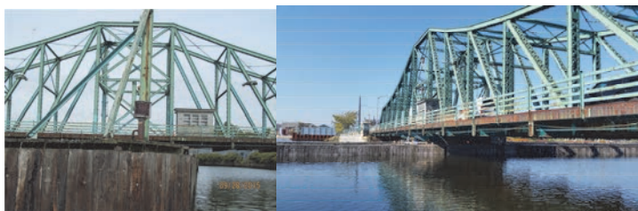
Grand Street Bridge in October 2015 (Pier 1- Right Side) and October 2016.
