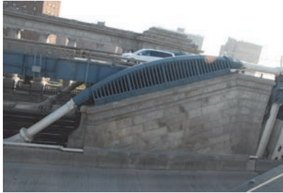
Manhattan Bridge Saddle. (Credit: Jagtar Khinda)
