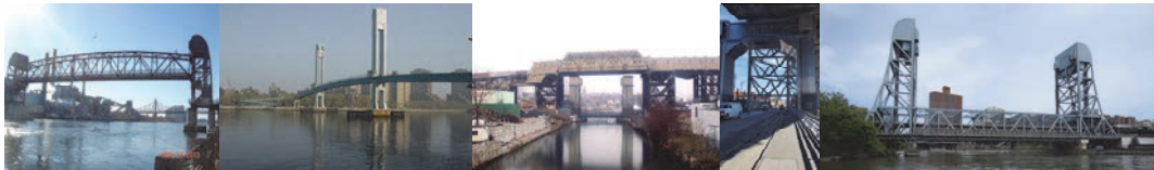
Lifted Roosevelt Island Bridge. (Credit: NYSDOT). Wards Island Pedestrian Bridge. Ninth Street Bridge. (9th Street Credits: Bojidar Yanev and Roly Parroco) Broadway Bridge.
