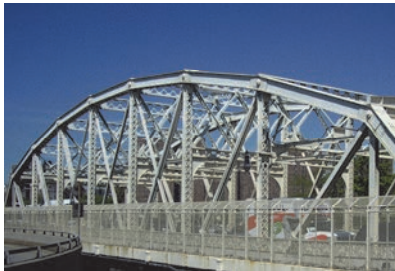
Macombs Dam Camelback Truss.
