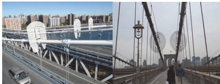
Suicide Gates on the Cables of the Manhattan (Credit: NYSDOT) and Brooklyn Bridges.
