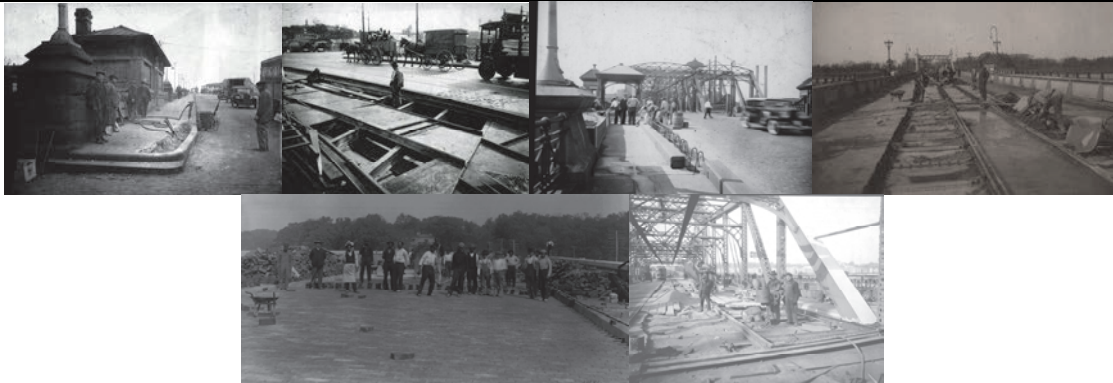
Willis Avenue Bridge Curbing and Road Repair in the Early 1920's. Madison Avenue Bridge - Constructing New Guardrail in September 1934. Concreting on City Island Bridge in 1912 and Shore Road in 1908. University Heights Bridge Roadway Repair in 1923.
