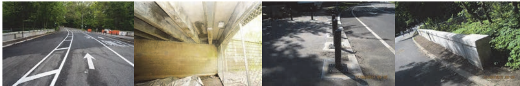
East Drive Bridge over Bridle Path After Construction.
