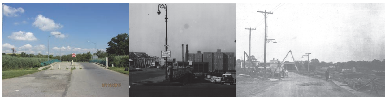
Boathouse Bridge over Aquacade Lake in 2017. (Credit: NYSDOT) Madison Avenue Bridge Posted Weight Restriction in Effect in 1959. Eastchester Temporary Bridge – Posted Weight Restriction in 1920.
