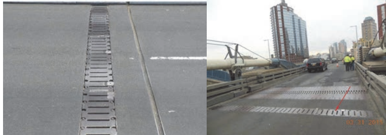
Manhattan Bridge Trench Drain.
