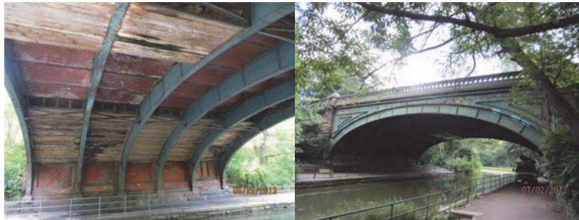
Hill Drive Bridge Span 2 Pier 1 End Face in 2013. View of Bridge in 2012. (Credit: NYSDOT)
