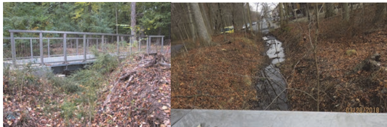
Springville Greenway Pedestrian Bridge over Freshwater Wetlands.
