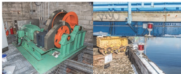
December 2017: Touch-Up Painting on Carroll Street Bridge Machinery. Pier Lights.
