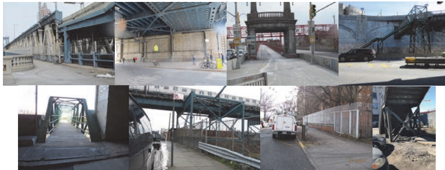
Winter Monitoring Locations: Manhattan, Williamsburg, and West 155 th Street Pedestrian Bridge. Fire Hazard Locations: Glenmore Avenue and Ocean Parkway Bridges Over LIRR Bay Ridge, and 51 st Avenue Pedestrian Bridge Over LIRR.
