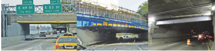
Retro-reflective Material Improves Visibility of These Low Vertical Clearance Bridges: East 60 th Street Bridge Over FDR Drive and Westchester Avenue Bridge over Hutchinson River Parkway. Vertical Clearance Beam at Span 53, Southbound Roadway of the Promenade over the FDR Drive. (FDR Credit: NYSDOT)
