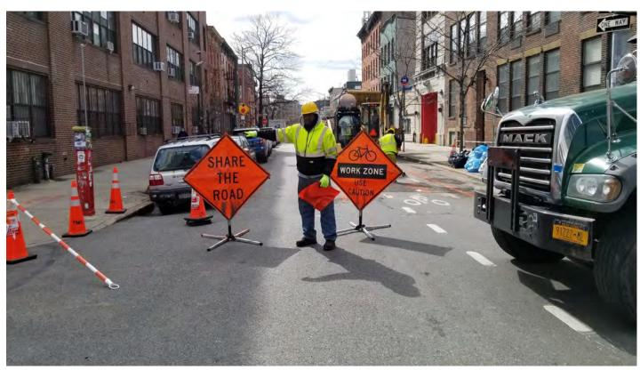
The signage indicates one direction, but the flagger is directing cyclist to perform a different maneuver. Also, signage requires better placement.
