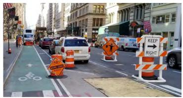
In both instances, the signage is generally placed in advance of the work zone and not blocking the bike lane, however, the signs need to be elevated.
