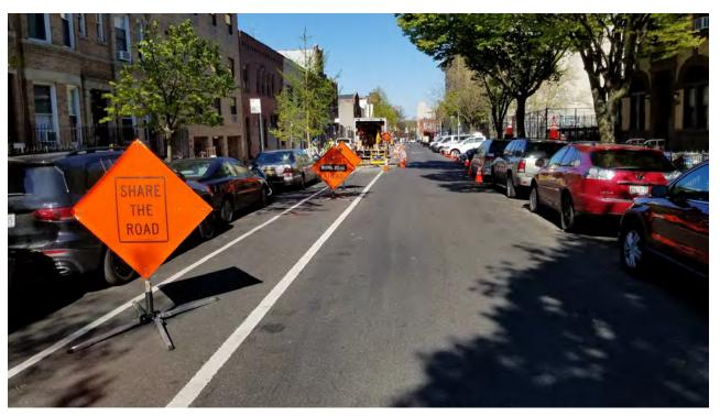
First sign is incorrectly place. It's also blocking the bike lane when it should be within the parking lane
