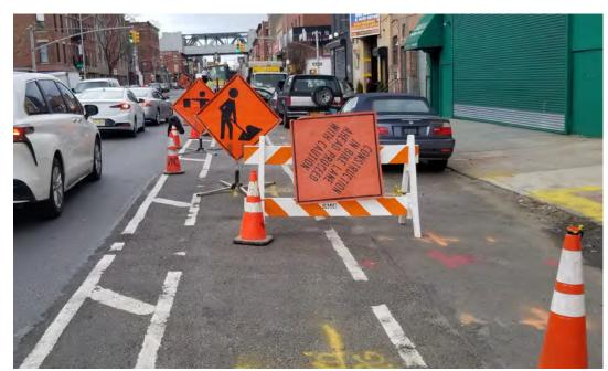
Sign is illegible due to its poor orientation.
