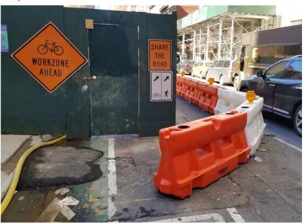
Work zone ahead sign is place at the work zone. The bicycle and pedestrian signage is confusing about where to go, To further confuse the situation is the Share the Road sign.
