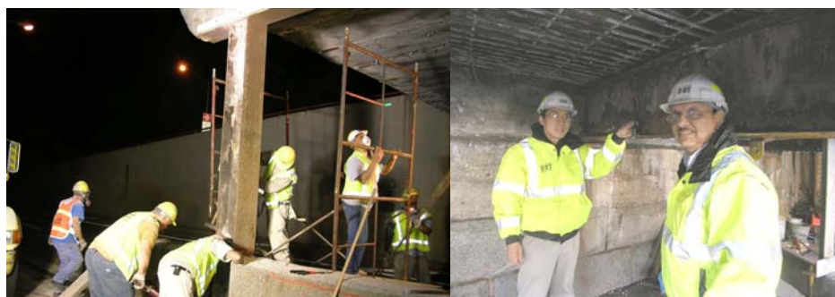
Red Flag Repairs at the Houston Street Bridge over the FDR Drive. (Credit: Hany Soliman) Assistant Civil Engineer Andrew Hoang and Civil Engineer Rajendra Pandya Measuring the Section Loss of the Bottom Flange of A Floor Beam, Utilizing a Digital Caliper.
