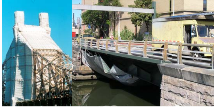
Queensboro Bridge Containment. (Credit: Peter Basich) Preventing Paint From Falling Into the Dutch Kills under the Hunters Point Avenue Bridge. (Credit: Sergiy Parayev)
