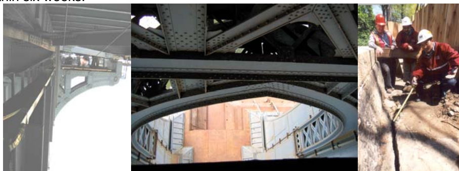
Flag Engineers Inspecting a Red Flag (Floor Beam Web) on the Tower Structure of the Manhattan Bridge. Closeup of the Location. (Credit: Bojidar Yanev) Flag Engineers Inspecting a Red Flag on the Central Drive Bridge over Transverse Road #1-- the West Fascia Had a Long Crack Running From the South Abutment Wall to the North Abutment Wall. (Credit: Peter Basich)
