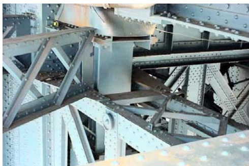
Truss Bearing on Manhattan Bridge. (Credit: NYSDOT)
