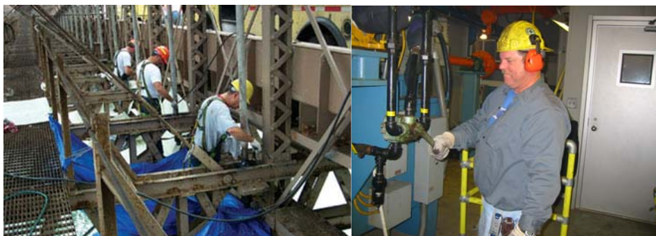
Maintenance Crew Conducting the Annual Cleaning and Lubrication of the Solid Rod Suspenders Spherical Bearings on the Brooklyn Bridge. (Credit: Anatoly Orlov) Oiler T. McAuliffe at the 9 th Street Bridge. (Credit: Vera Ovetskaya)
