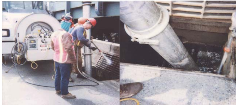
Cleaning Catch Basins on the Manhattan Bridge
