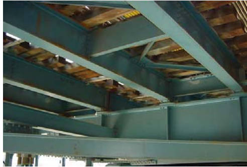
South Transit Floorbeams, Stringers, and Bracing Members on the Manhattan Bridge. (Credit: NYSDOT)
