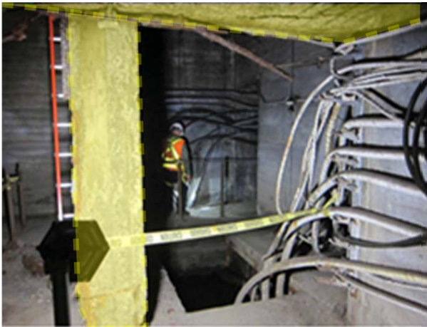
Column & beam repair
