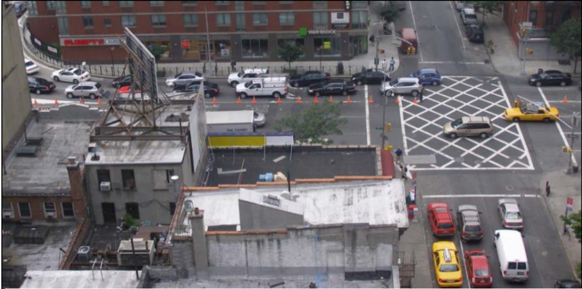
Figure 2.3.2: West 37 th Street, Looking West towards 9 th Avenue
