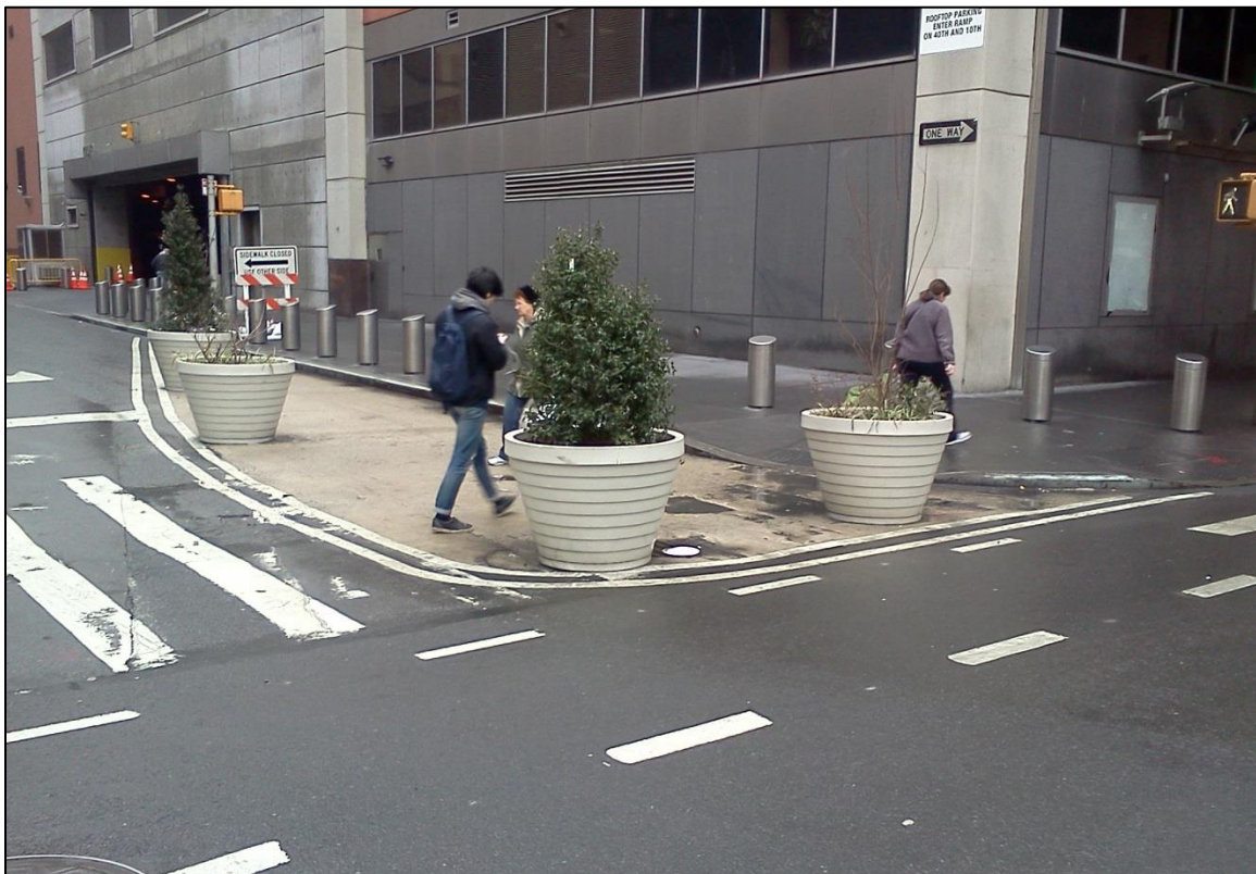
Figure 3.9.3: Curb Extension at Southeast Corner of West 41 st Street and 9 th Avenue
