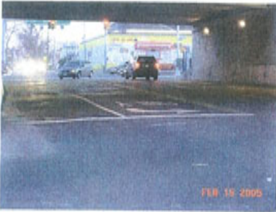
Narrowing of sidewalks to provide an additional lane. New configuration 2 northbound and 3 southbound lanes
