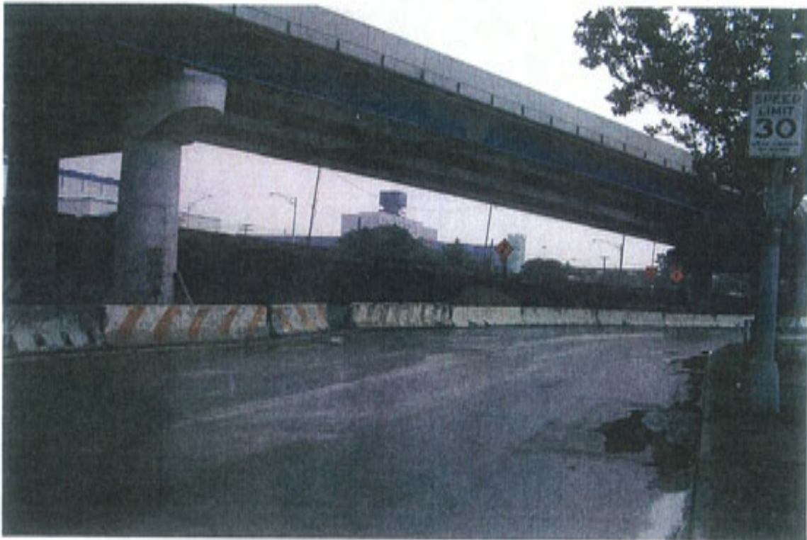
End of the proposed U-turn, traffic from U-turn SB SR and from the expressway NB SR
