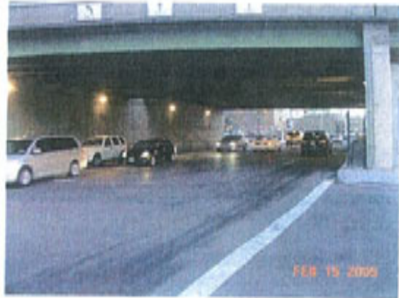
Narrowing of sidewalks to provide an additional lane. New configuration 2 northbound and 3 southbound lanes
