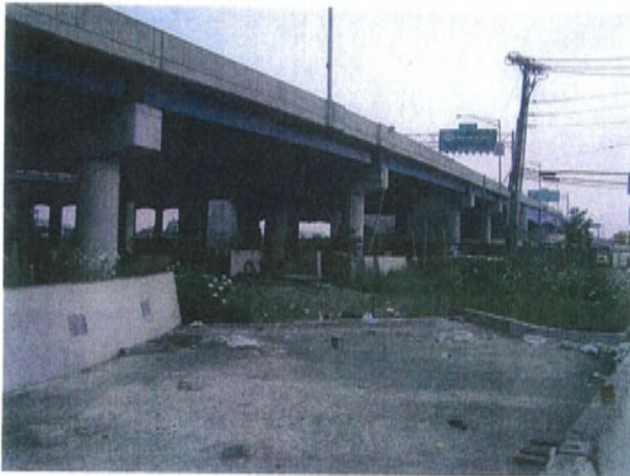
Site of proposed U-turn from southbound SR to northbound SR
