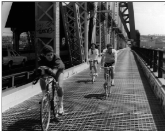
Queensboro Bridge bicycle path
