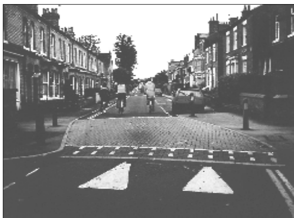
Speed table used to slow vehicular traffic on a residential street in York, England.
