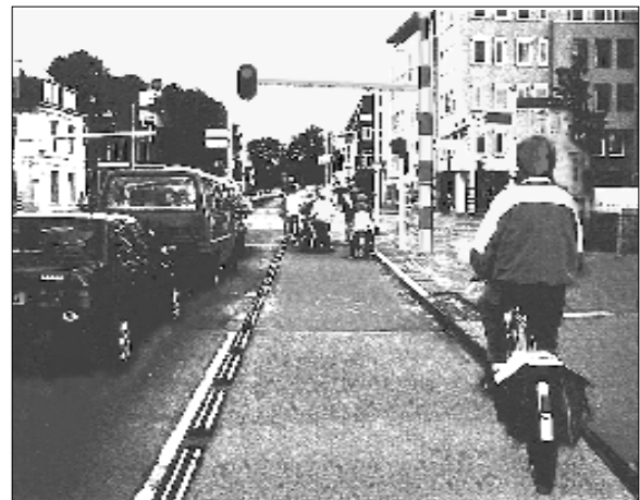
Bicycle lane in Frankfurt, Germany separated from motor vehicle traffic by a series of rubberized curbs, anchor bolted into the street pavement.
