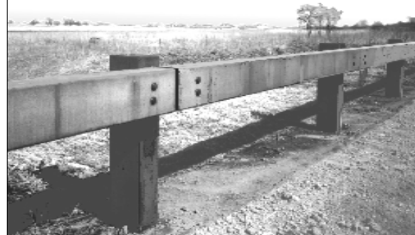
Steel barrier rail installed along the perimeter of Marine Park, Brooklyn.
