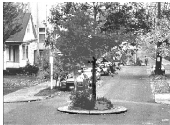
Traffic circle used to reduce through vehicular traffic while allowing local access in a residential neighborhood of Seattle.
