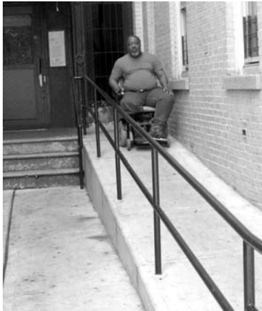
A case brought before the Commission resulted in the installation of a ramp for a tenant.
