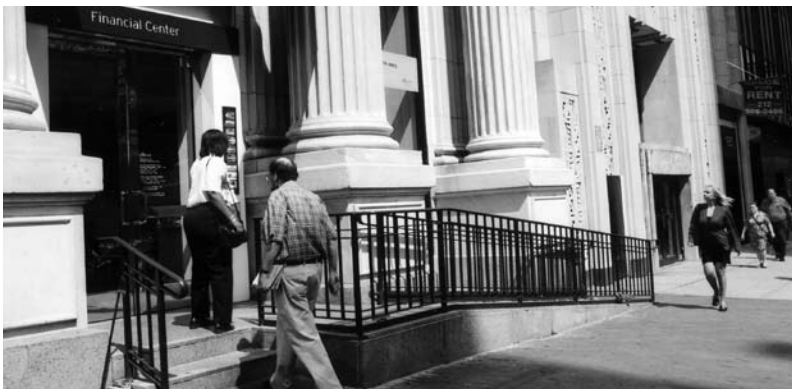
A major bank implemented changes to many of their branches to accommodate persons with disabilities.
